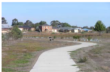
Recently completed shared path along Serendip Creek which will eventually connect the town centre to the You Yangs.
