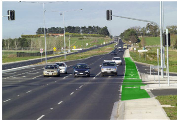
Figure 9: Back of Kerb Bicycle lane.
