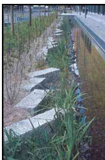
Example of a swale drainage system
