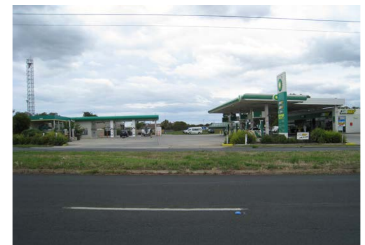
BP service station on the Bellarine Highway
