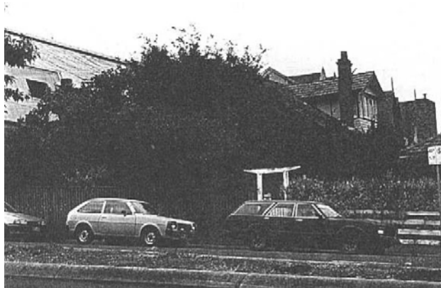
Dwelling, 299 Moorabool Street, 1995. Source: Helen Lardner Conservation & Design, City of Geelong Urban Conservation Study Locally Significant Sites, vol.4a, 1995.
