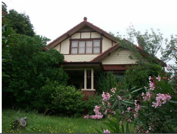
Front (west) elevation, March 2011.
