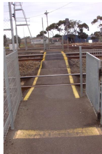
Abutment of surface and width of space limit access
