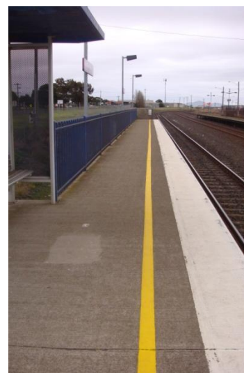
Lack of tactile ground surface indicators
