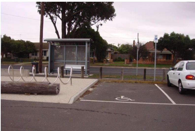
Lack of appropriate line marking and connections
