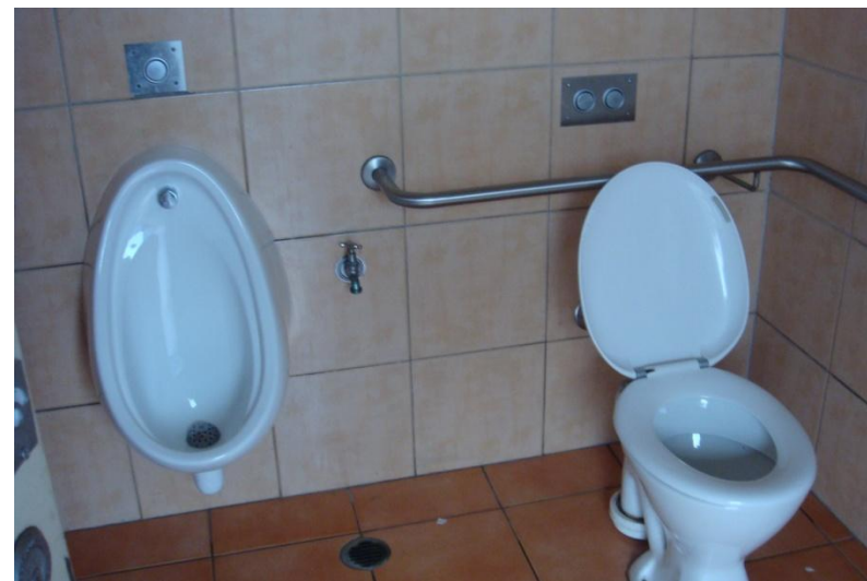
Location of urinal limits pan circulation space
