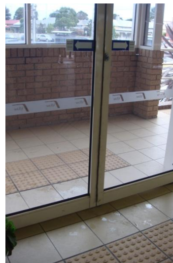
Inappropriate contrast strip on glazing
