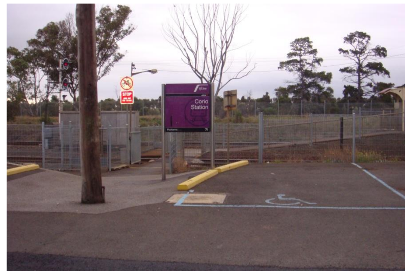
Limitations to parking and walkway
