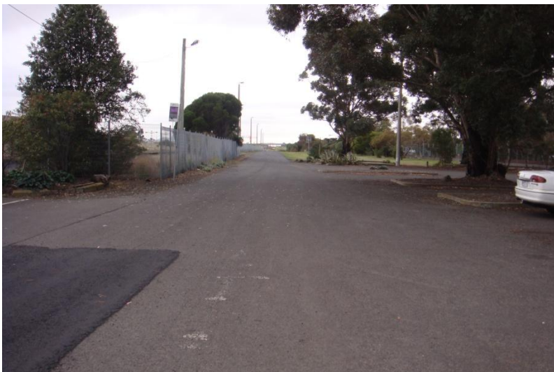
Lack of continuous access path of travel from allotment boundary
