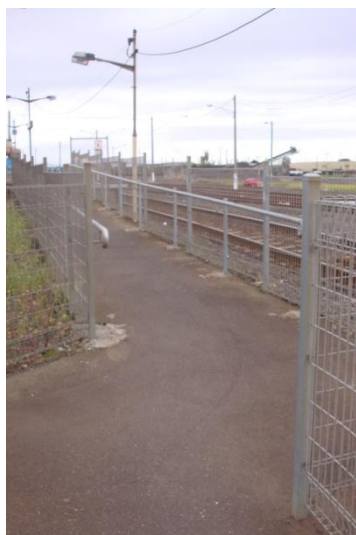
Lack of appropriate kerbs and contrasts
