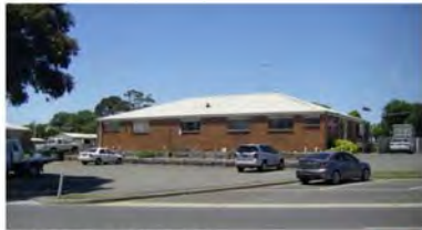
THE PHOTO EXISTING CONDITION
