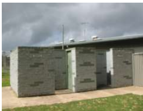
Photo 23: Public toilets at Cricket Club
