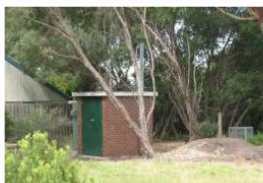
Photo 29: Barwon Water pumping station
