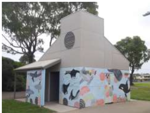
Photo 21: Public toilets on Sheepwash Road
