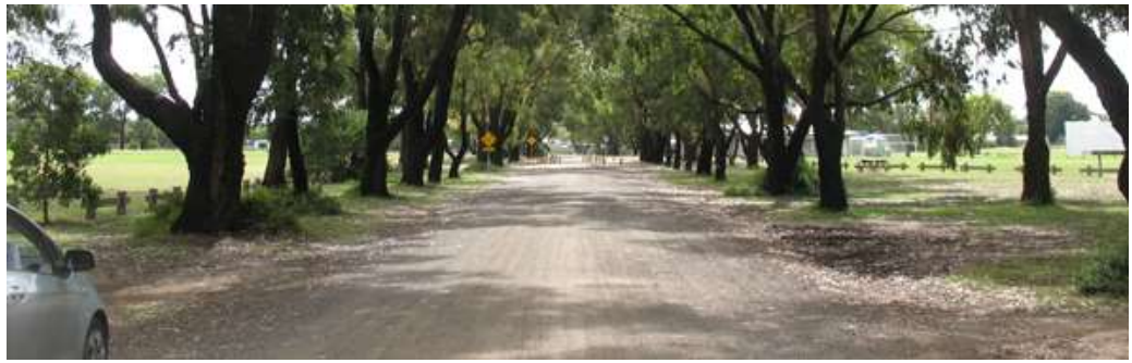
Photo 31: Hitchcock Avenue extension
