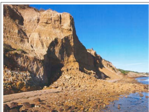
Photo 4 Cliff erosion at Beacon Point
