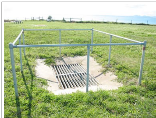
Photo 18 Existing drain pit
