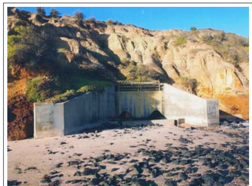
Photo 19 Existing drain outfall at Beacon Point
