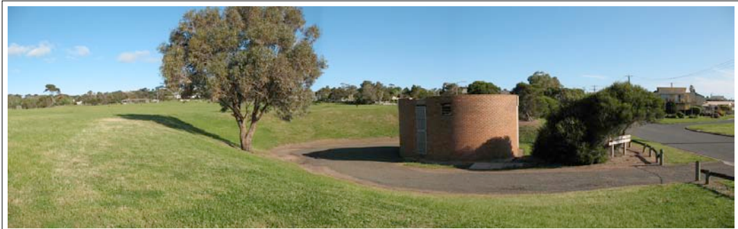
Photo 17 Barwon Water sewerage pumping station
