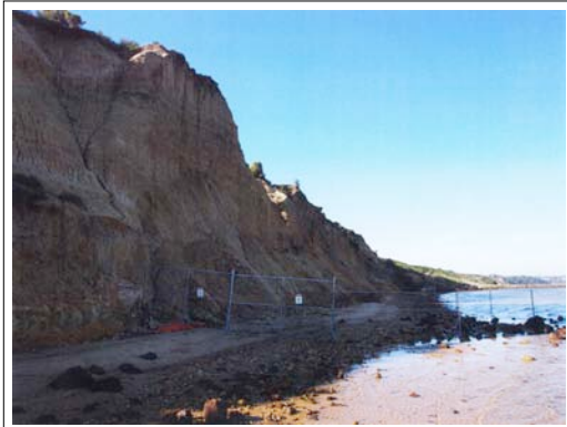
Photo 7 Restricted access due to cliff erosion
