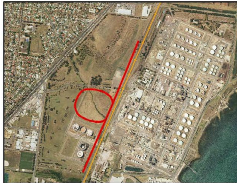
(5f) New rail loop to the west of the existing mainline rail track, bulk materials transfer solution to port required
