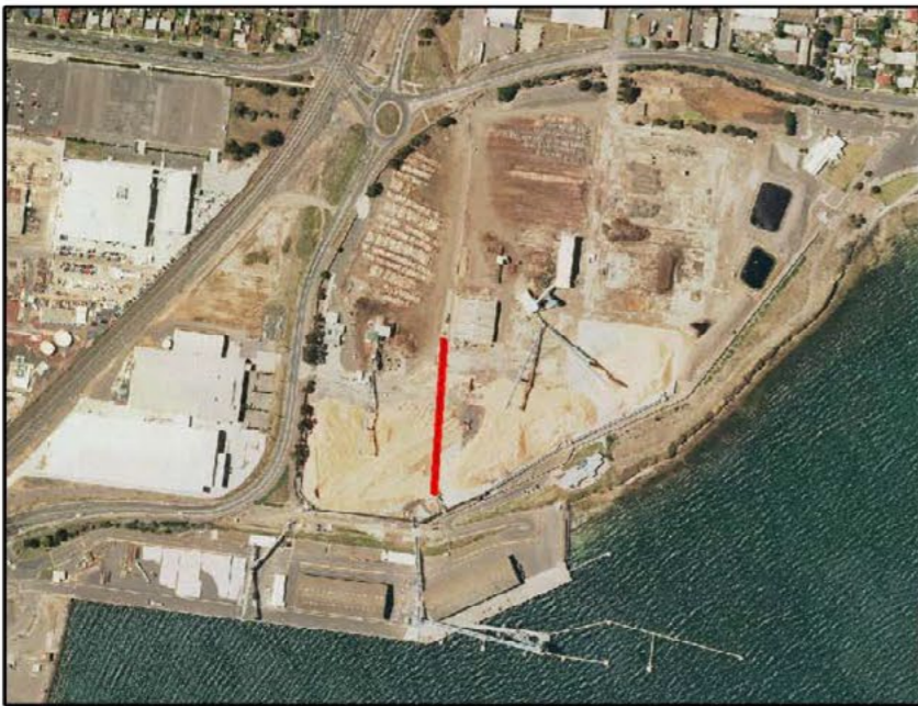
(5b) Midway siding extension.
