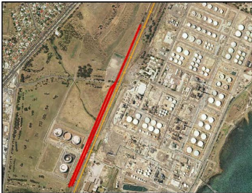
(5e) New siding extension to the west of the existing mainline rail tracks, bulk materials transfer solution to port required.
