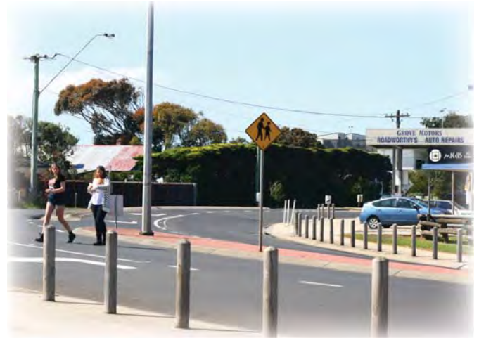
Figure 12: Existing sweeping bend on Hodgson Street - to be squared up under Phase 2 creating a new development site
