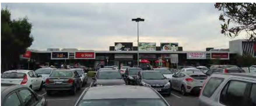
Figure 29 – Leopold Shopping Plaza located at the Bellarine Highway
