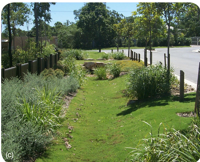
Figure 13 Selection of WSUD assets clockwise from top left (a) wetland (Grinter Reserve), (b) bioretention (Creekside Drive), (c) swale (Forest Lake), (d) sedimentation basin (Estuary Boulevard)
