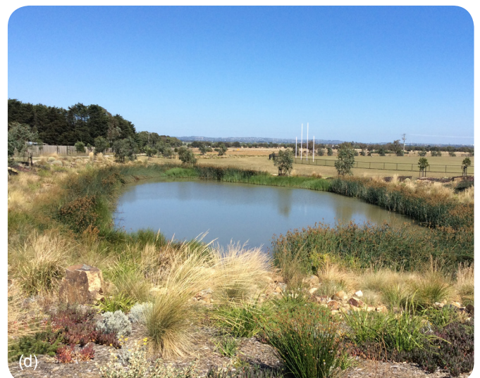
Figure 13 Selection of WSUD assets clockwise from top left (a) wetland (Grinter Reserve), (b) bioretention (Creekside Drive), (c) swale (Forest Lake), (d) sedimentation basin (Estuary Boulevard)
