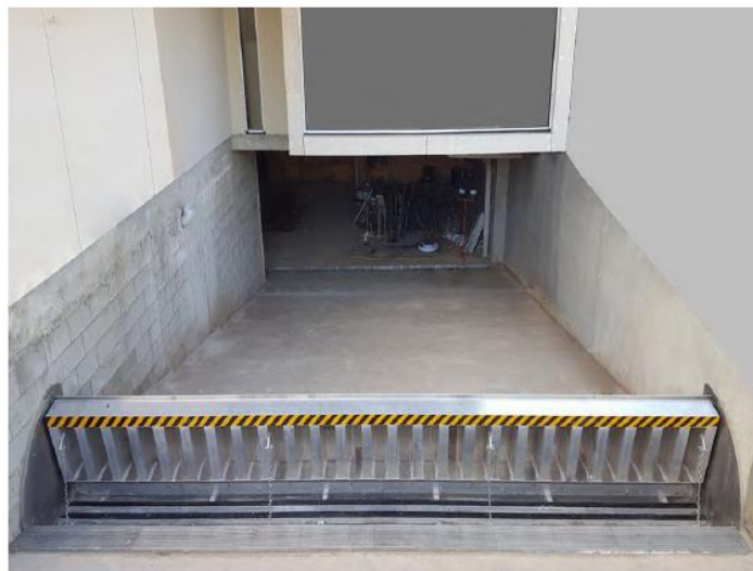
Figure 4-2 Example flood gate ( www.awmwatercontrol.com.au )
