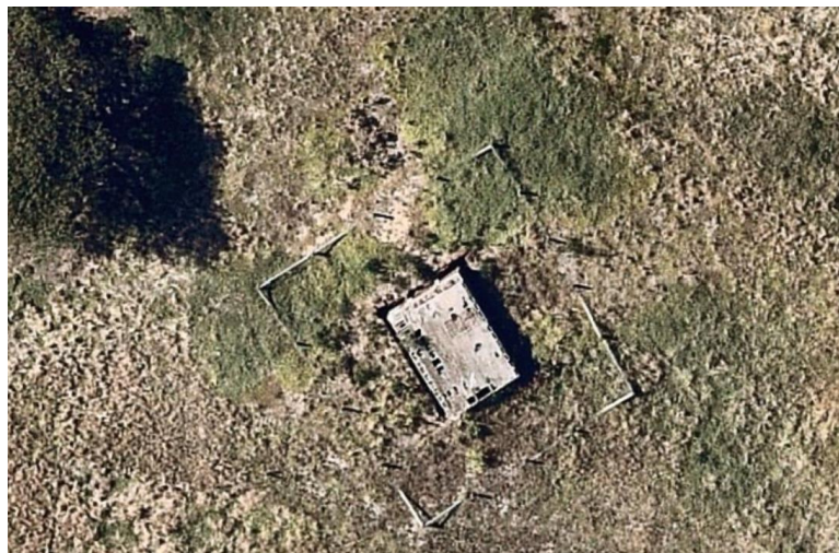
Aerial image, 20 January 2022 showing remnant former dairy outbuilding. Source: NearMap.
