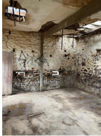
Former Dairy Outbuilding, interior, 2020.
