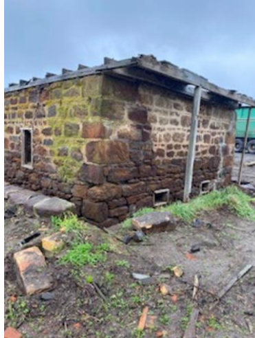
Former Dairy Outbuilding, west and south elevations, 2020, following removal of the roof. Source: Michael Burge, City of Greater Geelong.
