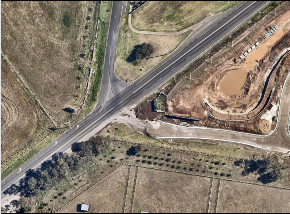
Figure 31 - Intersection of Point Richards Road with Portarlinton Road/Geelong Road. Source: Nearmap.
