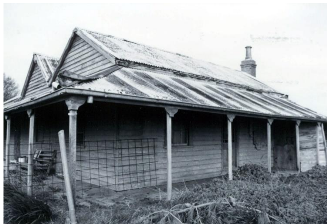
Lincoln's Farm, north-east corner of former dwelling, 1991. Source: Underwood.
