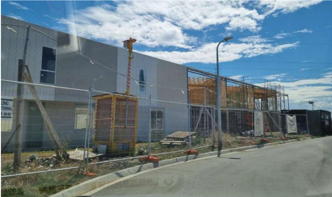
The 9 dwellings currently under construction
