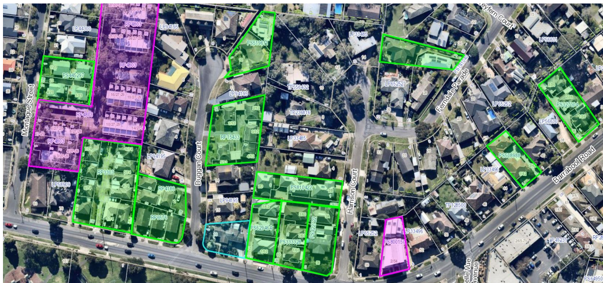
Image 8 – aerial imagery showing occurrence of infill development in proximity to subject site.
