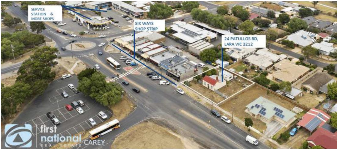
Image 5 – Taken from planning report submitted with application – aerial view of subject site and surrounding streetscape.
