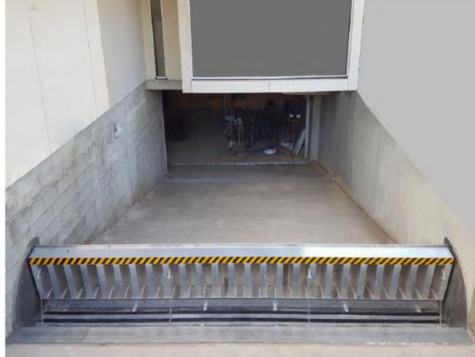
Figure 4-2 Example flood gate ( www.awmawatercontrol.com.au )
