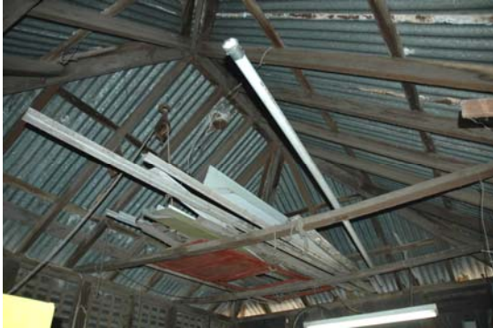
Photo 3.128: Interior, former Latrines Shed. Ceiling detail.
