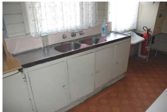
Photo 3.115: Interior, Kitchen. Detail of kitchen sink and cupboards, west wall.
