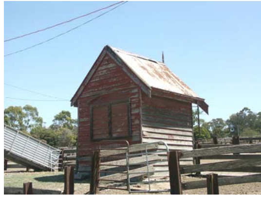
Photo 3.05: Former Gate Keeper's Cottage, north & east elevations.
