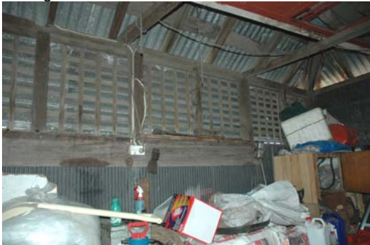
Photo 3.130: Interior, former Latrines Shed. View looking south showing early timber lattice wall screens with ripple iron cladding below.
