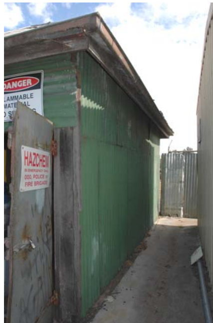
Photo 3.127: Former Latrines Shed, north elevation.
