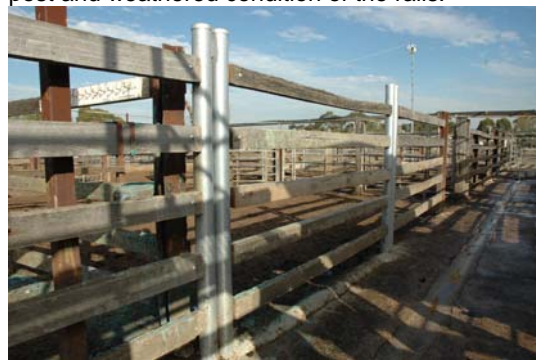
Photo 3.19: Detail of introduced round hollow steel posts and timber rail pen fence.
