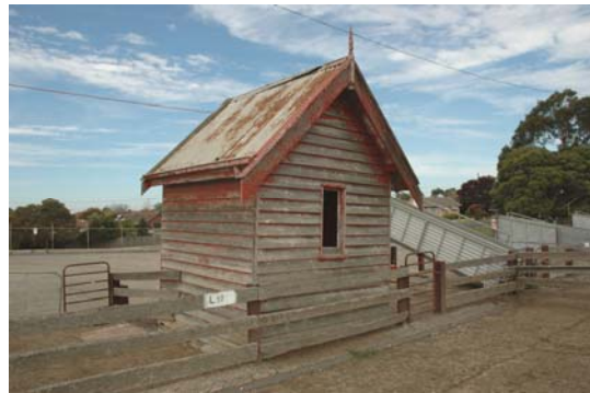
Photo 3.135: Former Caretaker's Cottage, west elevation.
