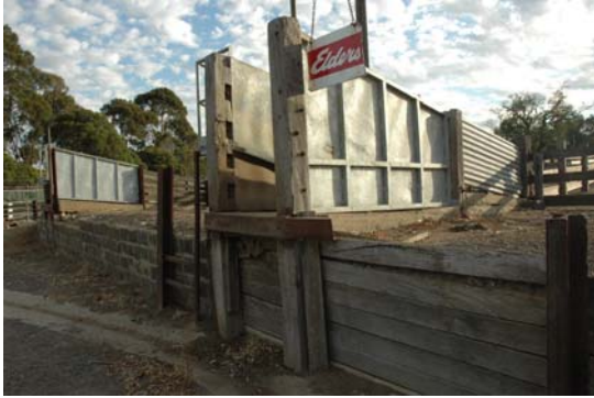
Photo 3.46: Ramp detail (sheep yard). The timber posts are early, but the metal panels and timber and bluestone retaining walls have been introduced.
