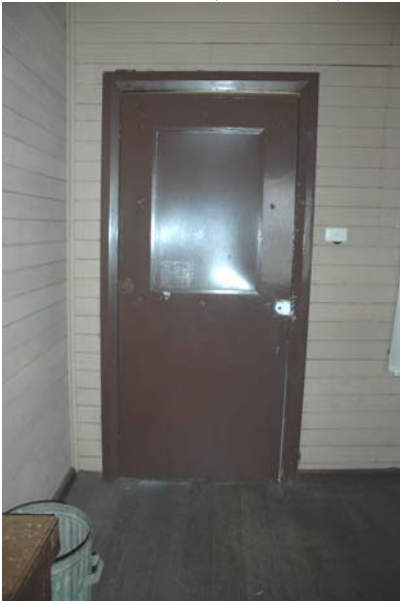
Photo 3.96: Interior, Bar Room. Detail of introduced flush panel timber door (east wall).
