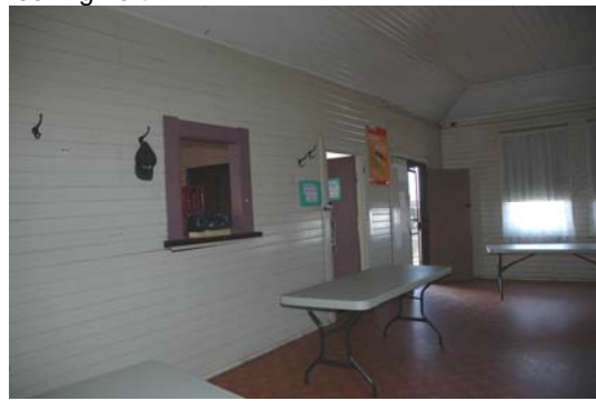
Photo 3.103: Interior, Refreshment Room, looking north-east.
