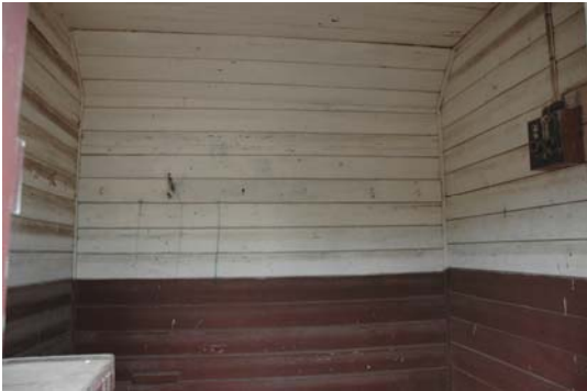
Photo 3.138: Interior, former Caretaker's Cottage. Wall detail.
