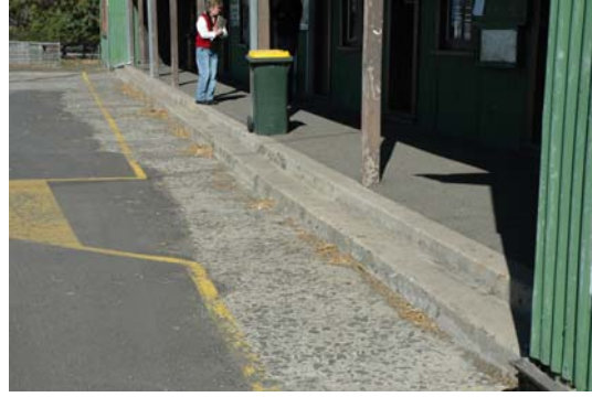
Photo 3.77: Market Offices building, east elevation. Detail of introduced elevated asphalt verandah floor and concrete steps.
