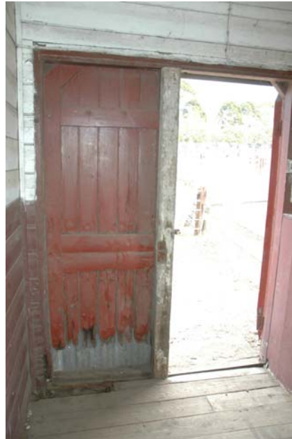
Photo 3.139: Interior, former Caretaker's Cottage. Door detail.
