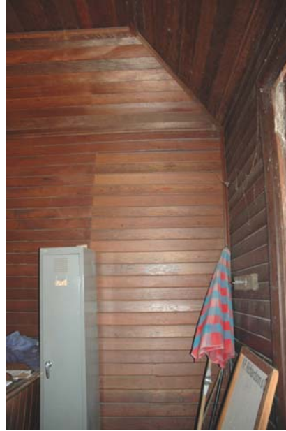
Photo 3.83: Interior, H.F. Richardson office. Detail of north wall showing blocked up door opening.
