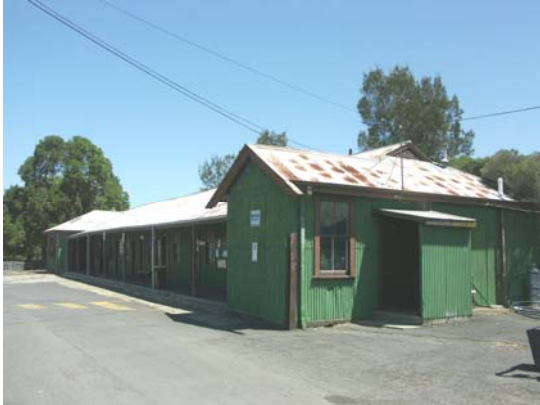
Photo 3.02: Market Office building, north & east elevations.
