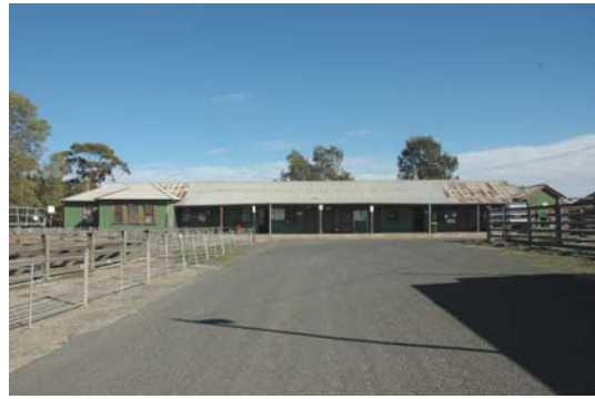
Photo 3.53: Market Offices building, east elevation, from the central thoroughfare.
