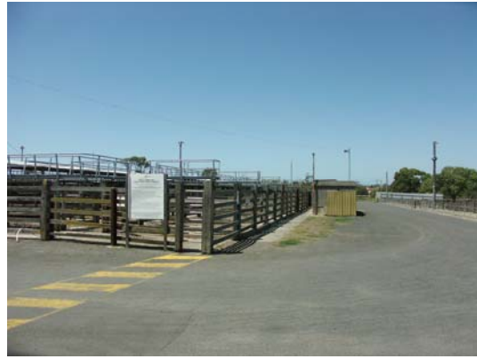
Photo 3.07: Cattle Yard, south-east corner.
