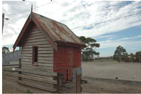
Photo 3.133: Former Caretaker's Cottage, south elevation.
