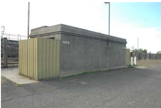
Photo 3.140: Toilet block, south elevation.
