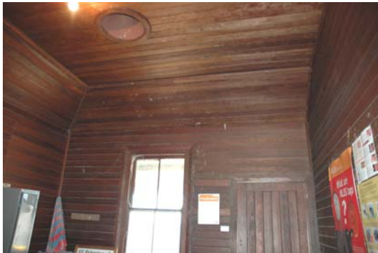
Photo 3.84: Interior, H.F. Richardson office. View looking east showing v-jointed timber ceiling and walls. Also note the early ceiling flue.
