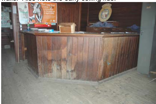
Photo 3.86: Interior, H.F. Richardson office. Detail of early timber sales bench.
