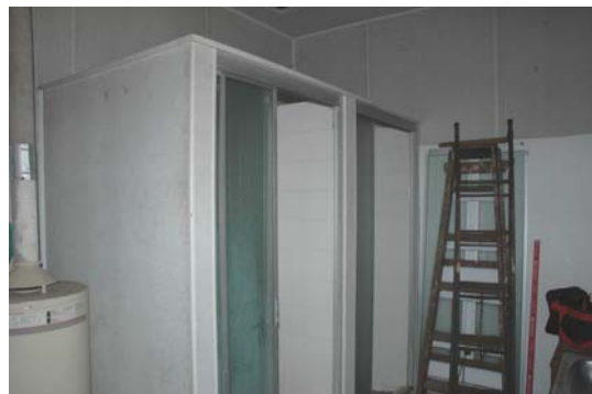
Photo 3.123: Interior, Staff Bathroom. Detail of introduced shower cubicles.
