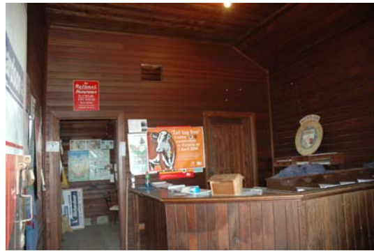
Photo 3.81: Interior, H.F. Richardson office, looking west. Note the early stained timber v-jointed ceiling and walls.
