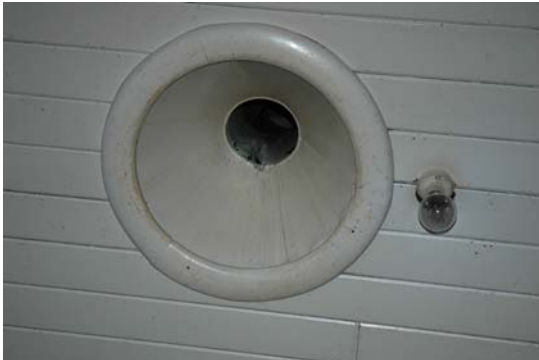
Photo 3.106: Interior, Refreshment Room, ceiling flue detail.
