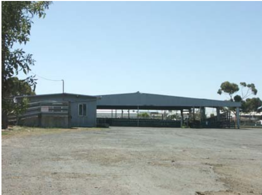
Photo 3.06: Pig Market Building & Office Building, south elevation.
