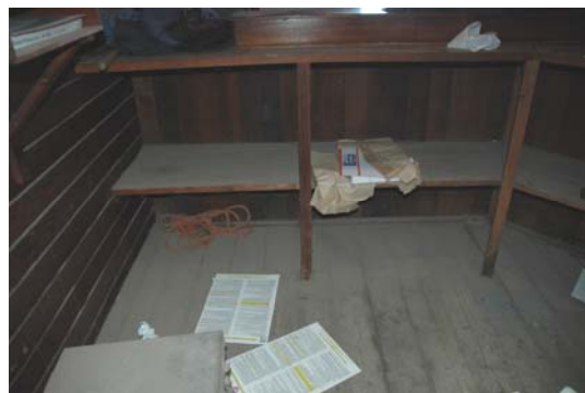
Photo 3.87: Interior, H.F. Richardson office. Detail of inner side of early timber sales bench showing the shelving.
