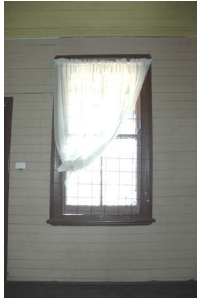
Photo 3.97: Interior, Bar Room. Window detail (east wall, north end).
