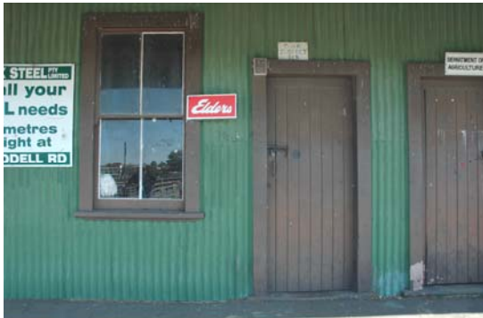
Photo 3.66: Market Offices building, east elevation. Office window and door detail (under verandah).
