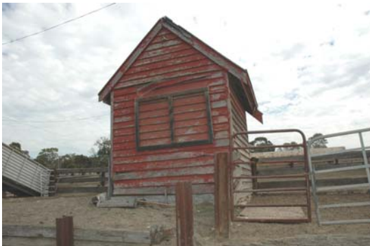
Photo 3.134: Former Caretaker's Cottage, east elevation.
