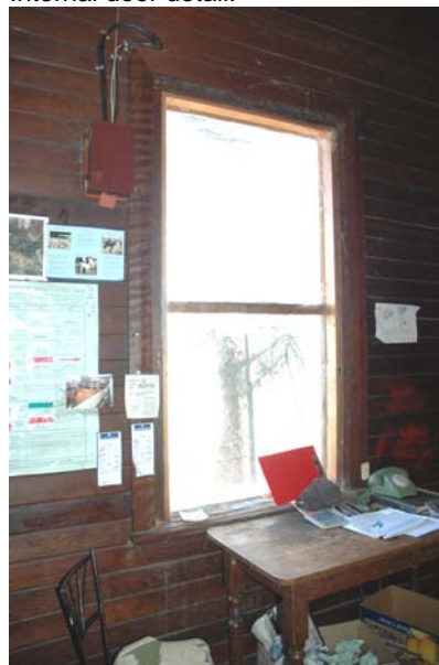
Photo 3.91: Interior, H.F. Richardson office. Window detail, rear office.
