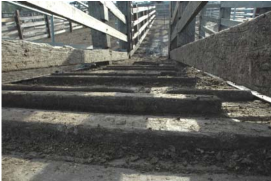
Photo 3.50: Detail of early timber ramp (cattle yard) showing sloped timber floor with raised battens. The floor has been reconstructed.
