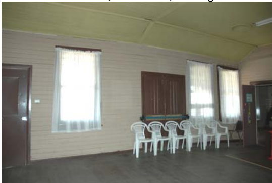
Photo 3.94: Interior, Bar Room, looking east.
