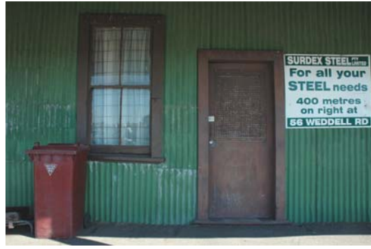
Photo 3.65: Market Offices building, east elevation. Office window and door detail (under verandah).
