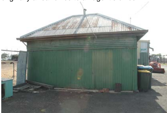
Photo 3.126: Former Latrines Shed, south elevation.
