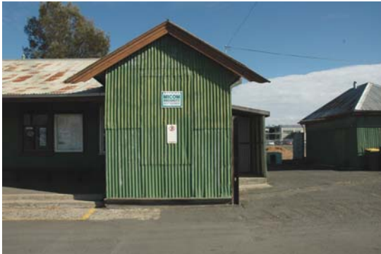
Photo 3.72: Market Offices building, east elevation. Detail of projecting office gable (north end of building).
