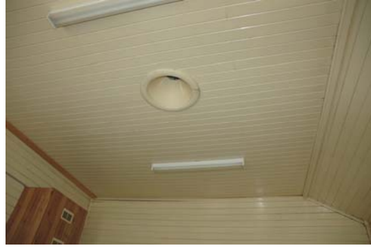
Photo 3.117: Interior, Kitchen. Ceiling detail looking east.
