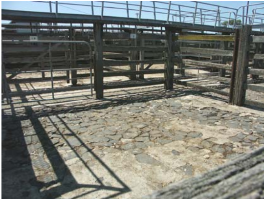
Photo 3.08: Detail of cattle pen no. 2. Note early timber posts & rails, & bluestone paving. Also note the introduced steel supporting post (right), being a recycled tram track.
