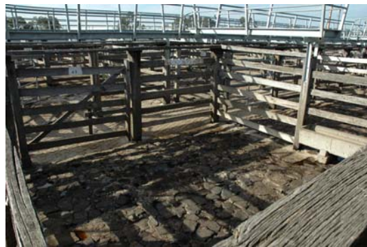
Photo 3.11: Detail of cattle pen no. 43. This pen is also substantially intact.
