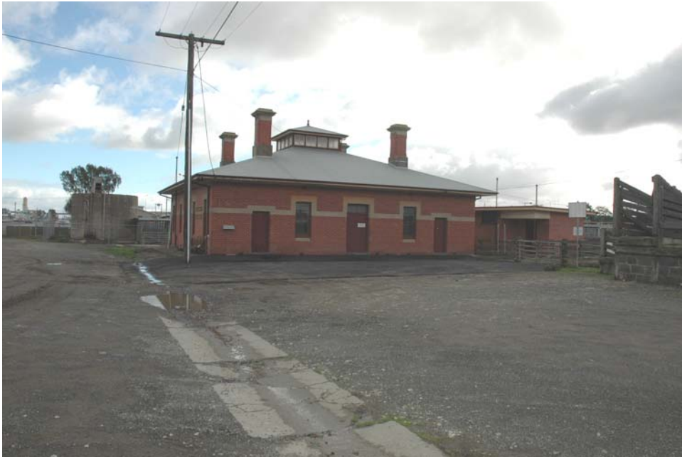
Figure 4.10: Market Offices building, Ballarat Sale Yards, 2007. Source: Wendy Jacobs.
