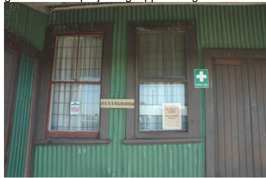
Photo 3.63: Market Offices building, east elevation. Window details (southern-most windows under verandah).
