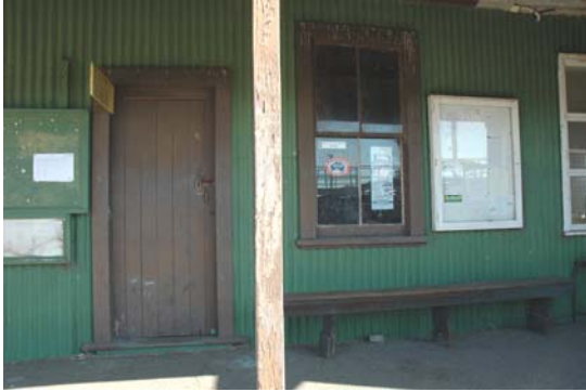
Photo 3.70: Market Offices building, east elevation. Office window and door detail (under verandah).
