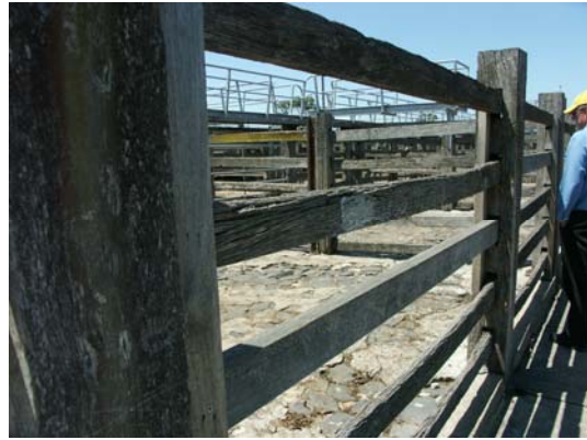
Photo 3.09: Detail of cattle pen no. 2 showing early square timber posts with narrow vertical slots taking the timber rails.
