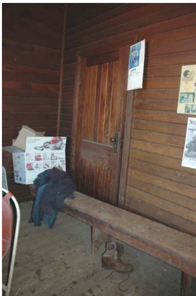
Photo 3.90: Interior, H.F. Richardson office. Detail of early door, wall and pew in rear office.
