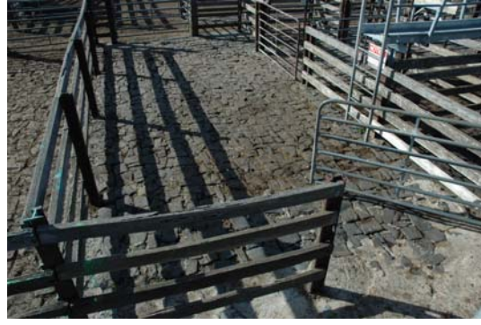
Photo 3.15: View of cattle pen showing bluestone paving, introduced steel posts (former tram tracks) and horizontal timber rails, together with introduced steel gates.
