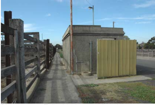
Photo 3.142: Toilet block, west elevation.
