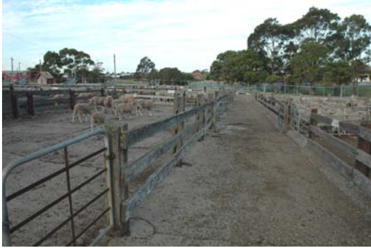
Photo 3.34: Detail of early timber posts with introduced timber rails bolts to the sides of the posts. These rails have replaced the original rails that were set in the vertical slots of the posts.
