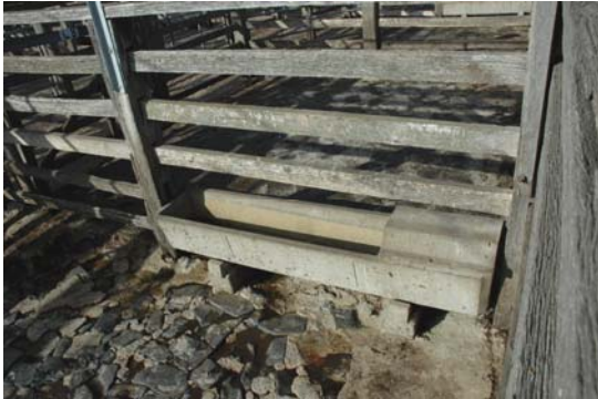
Photo 3.30: Detail of introduced concrete trough in cattle pen.
