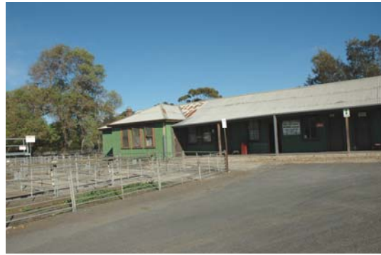
Photo 3.55: Market Offices building, east elevation (central and southern portions).
