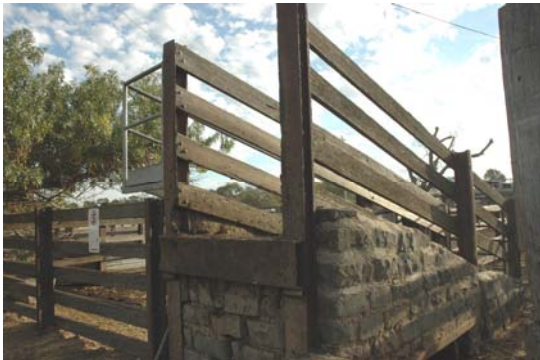
Photo 3.52: Detail of early (altered) ramp (cattle yard). Note the introduced steel posts (former tram tracks), timber rails and introduced bluestone base.
