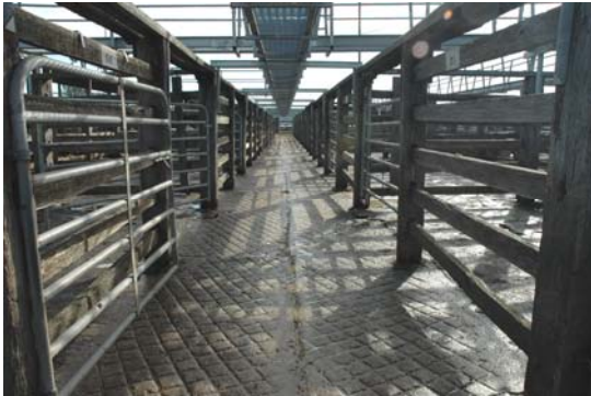
Photo 3.20: Detail of internal walkway showing central invert drain. The fibrous concrete paving has been introduced.
