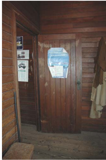
Photo 3.89: Interior, H.F. Richardson office. Internal door detail.
