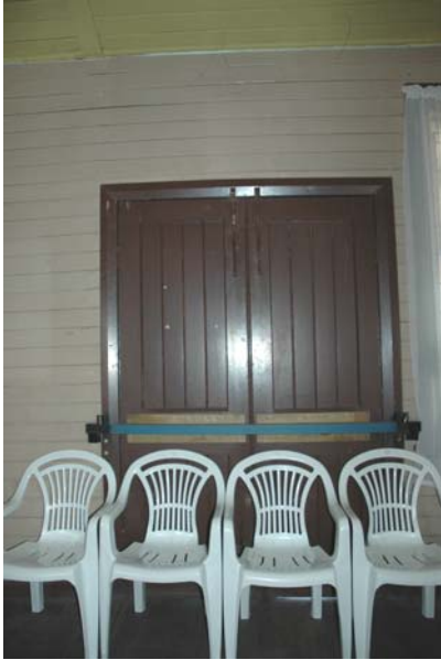
Photo 3.98: Interior, Bar Room. Detail of double door opening and v-jointed timber doors (east wall).
