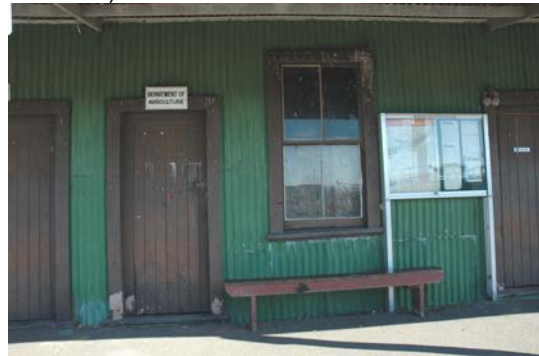
Photo 3.67: Market Offices building, east elevation. Office window and door detail (under verandah).
