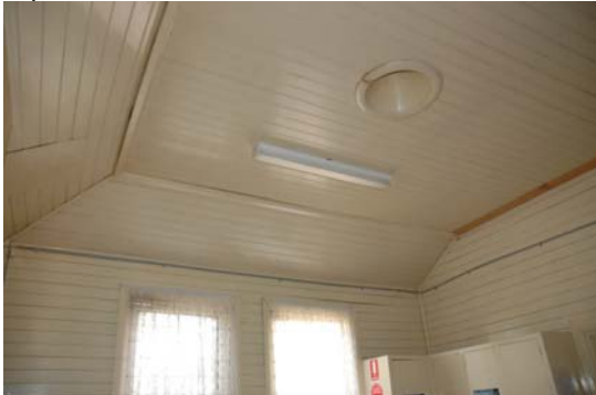
Photo 3.118: Interior, Kitchen. Ceiling detail looking north-west.
