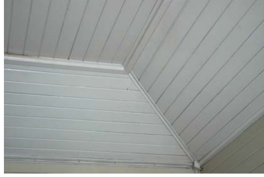
Photo 3.105: Interior, Refreshment Room, ceiling detail.
