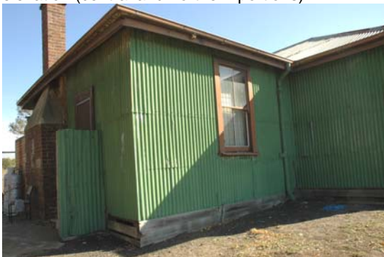
Photo 3.56: Market Offices building, east & south elevations (southern kitchen portion).
