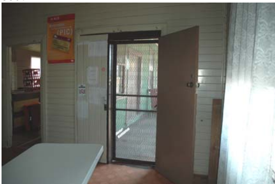
Photo 3.102: Interior, Refreshment Room. Detail of north external door opening & introduced flush panel timber door.
