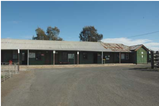
Photo 3.54: Market Offices building, east elevation (central and northern portions).
