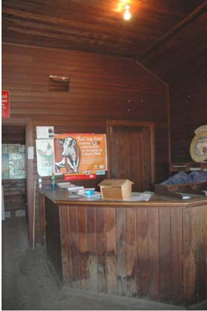
Photo 3.82: Interior, H.F. Richardson office. Note the v-jointed timber ceiling and the built-in sales bench.
