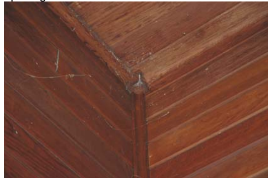
Photo 3.85: Interior, H.F. Richardson office. Detail of timber scotia mould ceiling cornice.
