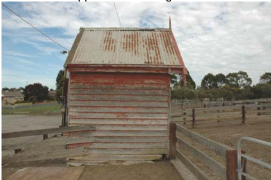
Photo 3.132: Former Caretaker's Cottage, north elevation.
