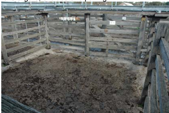
Photo 3.12: Detail of cattle pen no. 14. This pen is substantially intact. Note the early timber plank walks.
