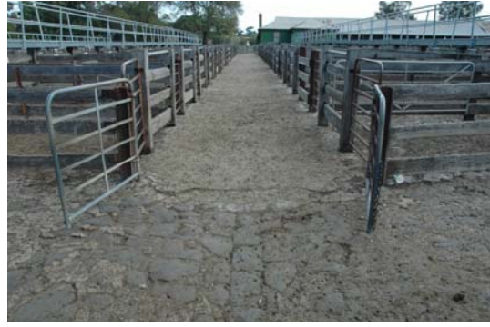
Photo 3.43: View of early bluestone paving (forming a spoon drain) and later concrete slurry finish in an internal walkway of the sheep yard.
