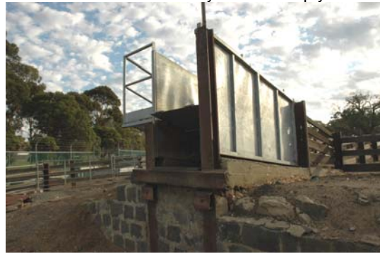
Photo 3.45: Ramp detail (sheep yard). This ramp has been introduced.
