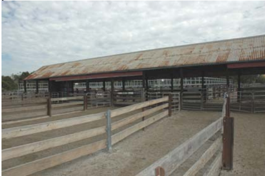
Photo 3.42: East elevation of the open shed in the sheep yard.
