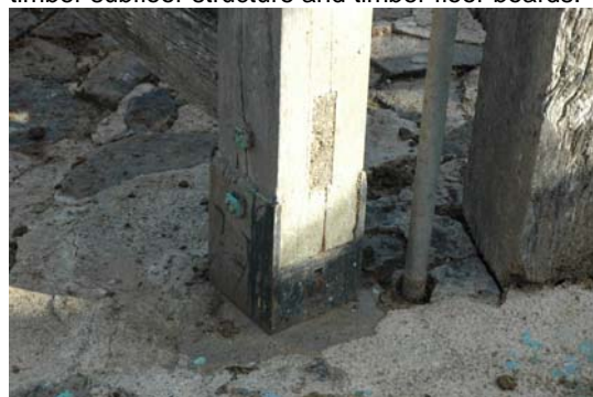
Photo 3.27: Detail of introduced steel stirrup gate post.
