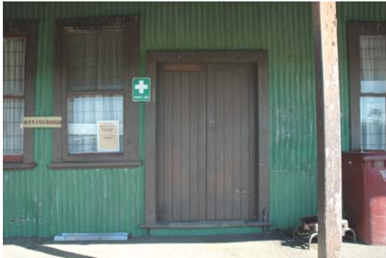
Photo 3.64: Market Offices building, east elevation. Detail of double door opening to Bar Room.
