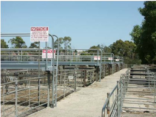
Photo 3.32: View of sheep yard looking south (from near the north-west corner). Note the introduced steel fencing and gates.
