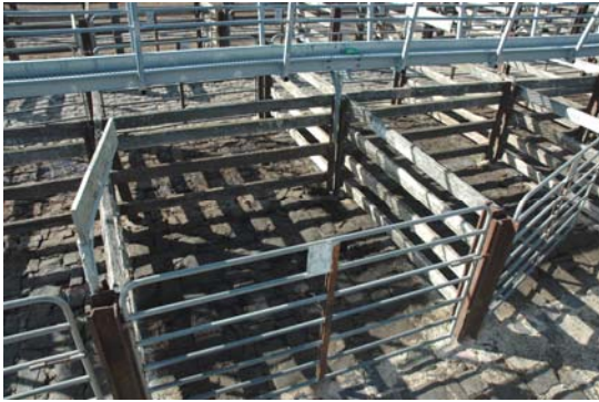
Photo 3.16: View of cattle pens showing introduced steel posts (former tram tracks), horizontal timber rails & steel gates. Note the early bluestone paving & the elevated introduced steel walk.
