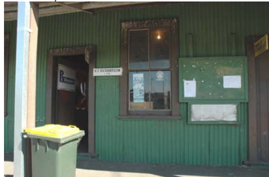
Photo 3.69: Market Offices building, east elevation. Office window and door detail (under verandah).
