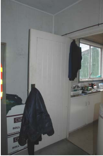
Photo 3.124: Interior, Staff Bathroom. Door detail (east wall). This door is an original v-jointed door in original location. The staff bathroom was originally a rear office to an agent's office.
