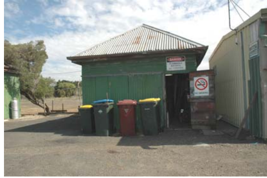
Photo 3.125: Former Latrines Shed, east elevation.
