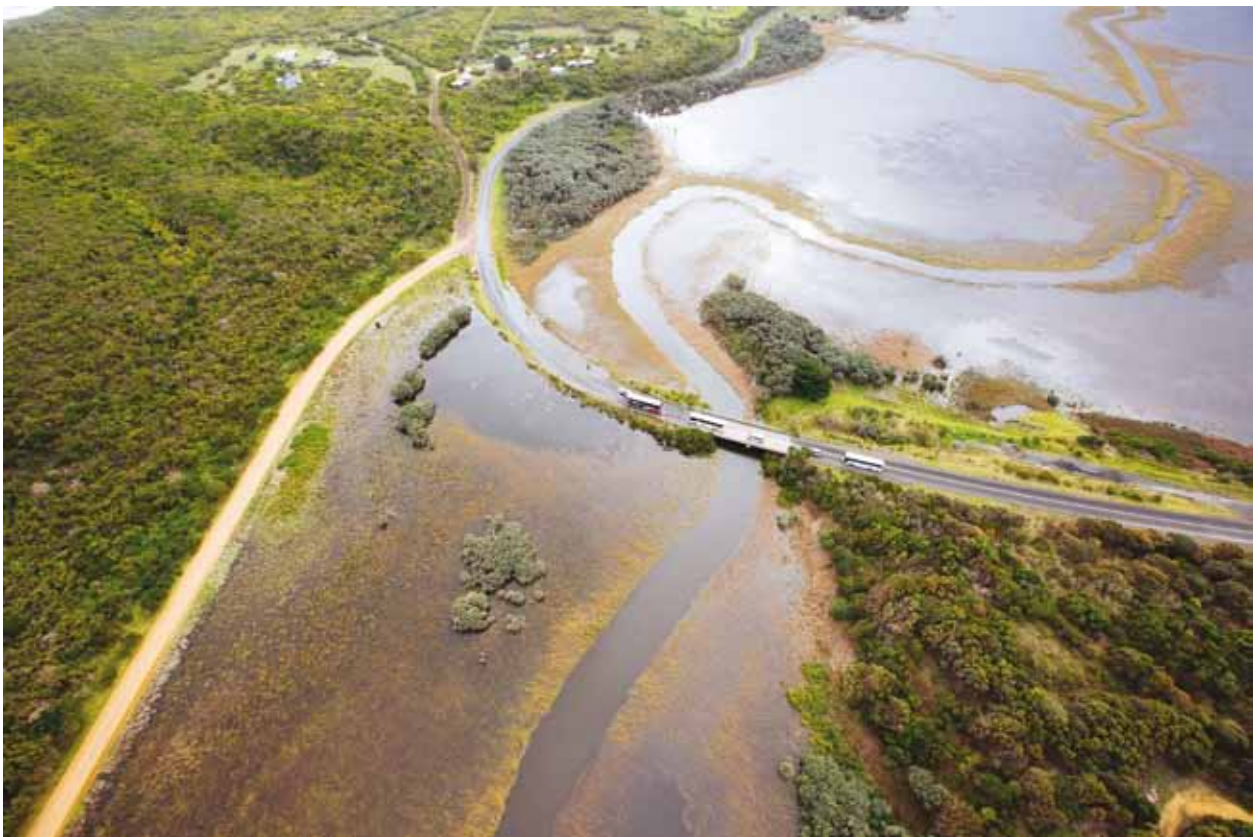
Flooding of the Gellibrand River estuary at Princetown during the May 2015 coastal storm surge showing inundation of the Great Ocean Road.
