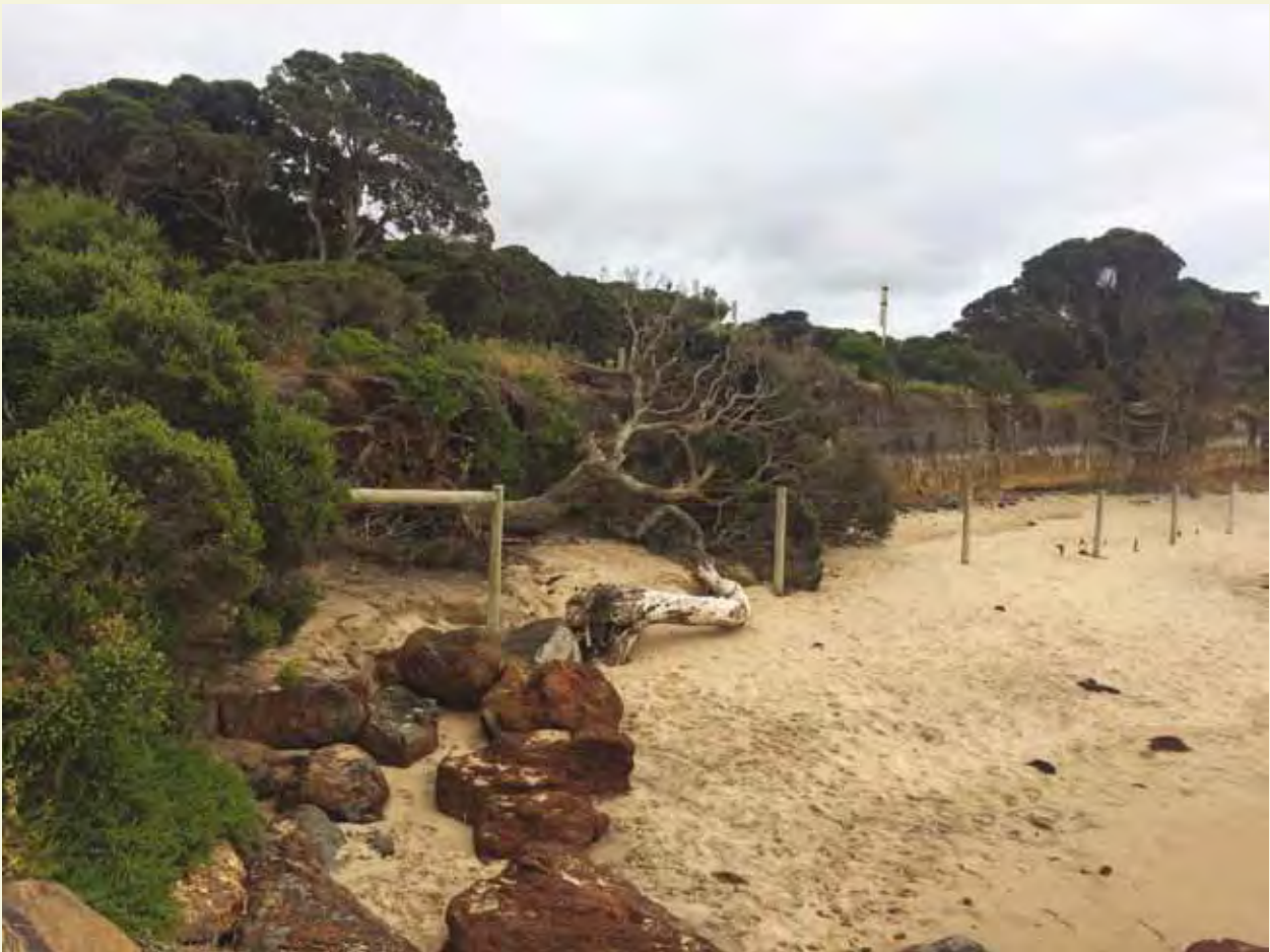
Erosion along Point Roadknight beach, Anglesea.
