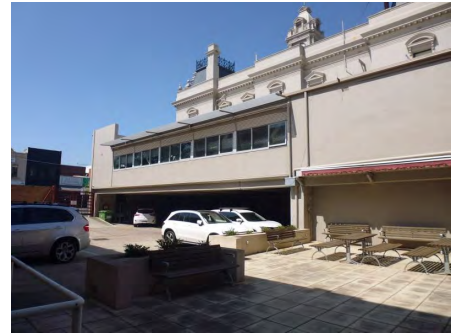
1939 addition on north elevation
