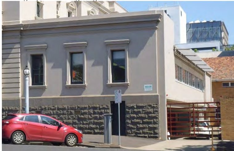
Addition on Gheringhap Street – mock Victorian street elevation
