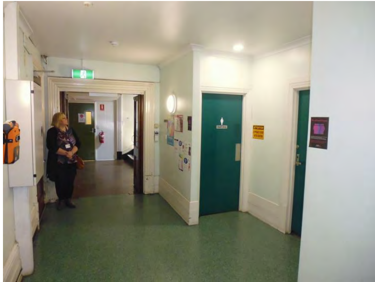
Rear ground floor, some original details but modern ceilings and partitions
