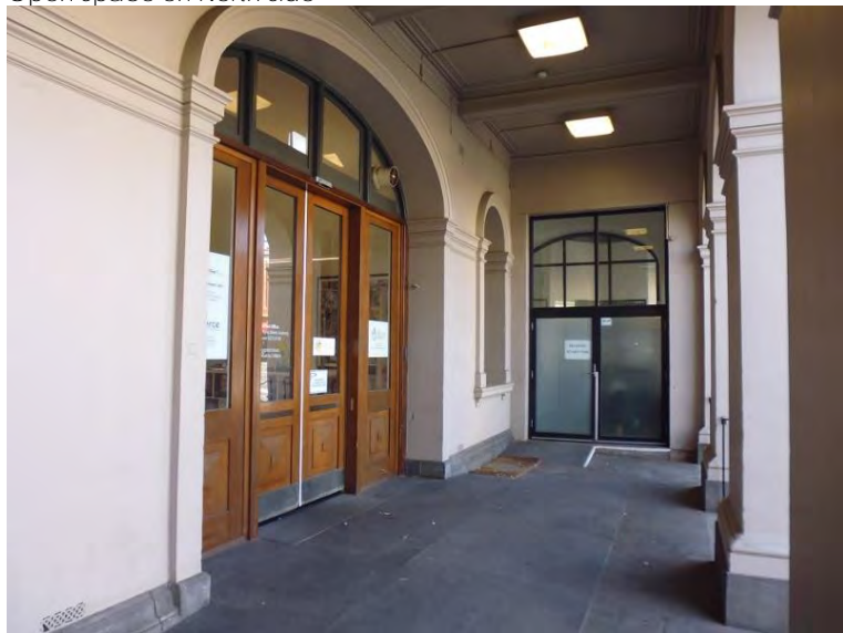
Ryrie Street Ground Floor Arcade
