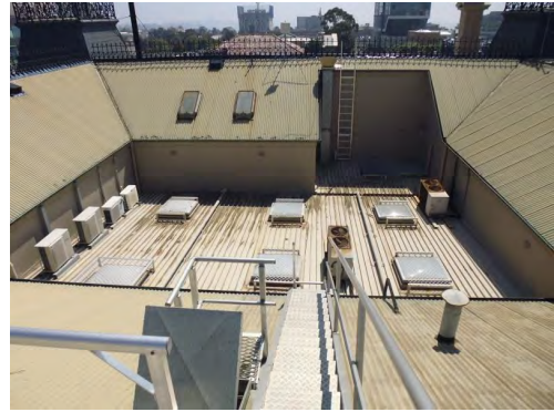
New internal roof
