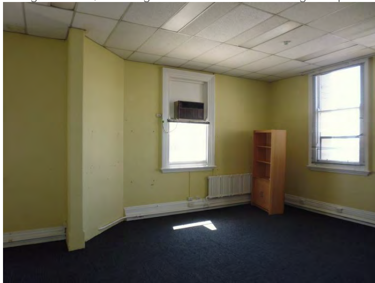
First Floor office, false ceilings, original walls removed, fireplace removed
