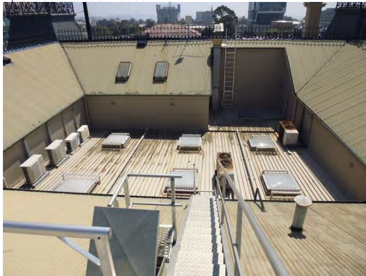
Roof - flat roof is an addition when the void was infilled
