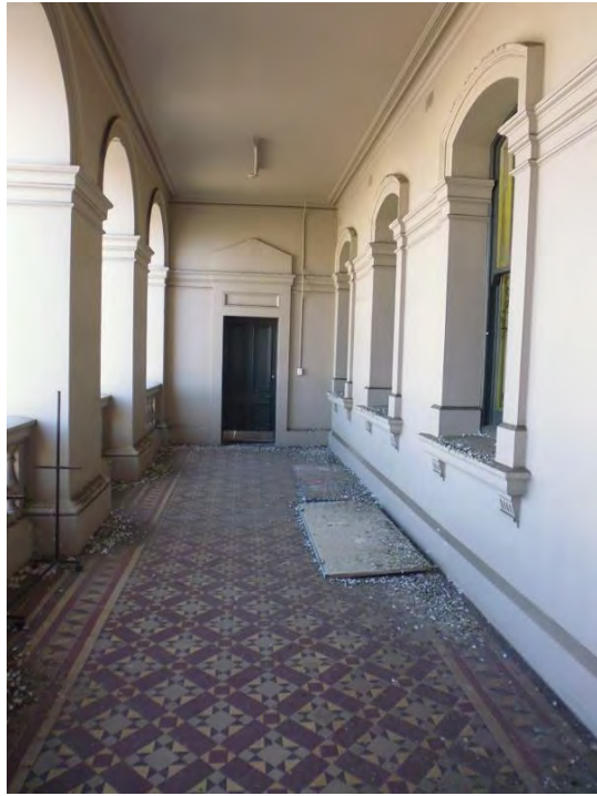
Ryrie Street First Floor Arcade
