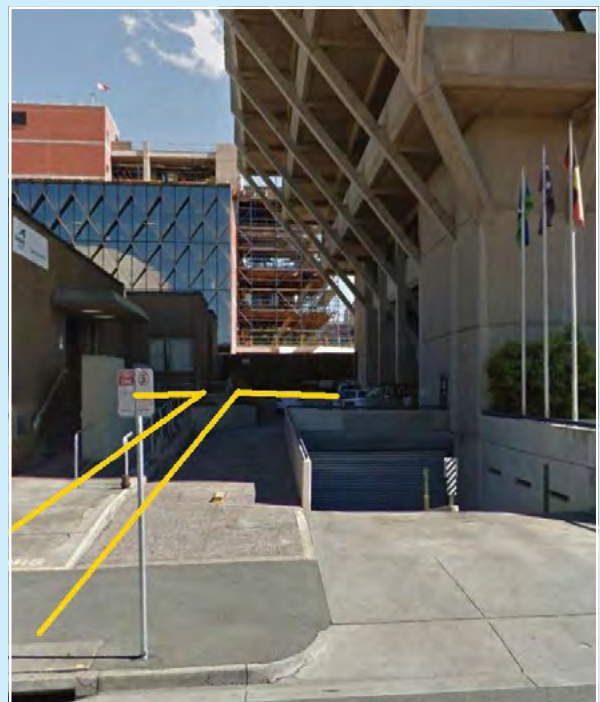
Figure 12. The potential alignment of a new Aitchison Place viewed from the north.
