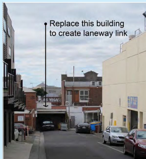
Figure 7. Potential link seen from the south along Market Street.
