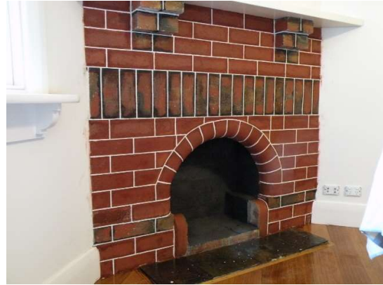
Fireplace, Geelong West, after restoration & tuckpointing. Source: Nat De-Palma.
