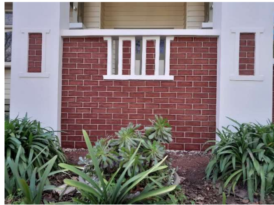
Verandah balustrade, Geelong, after restoration & tuckpointing. Source: Nat De-Palma.
