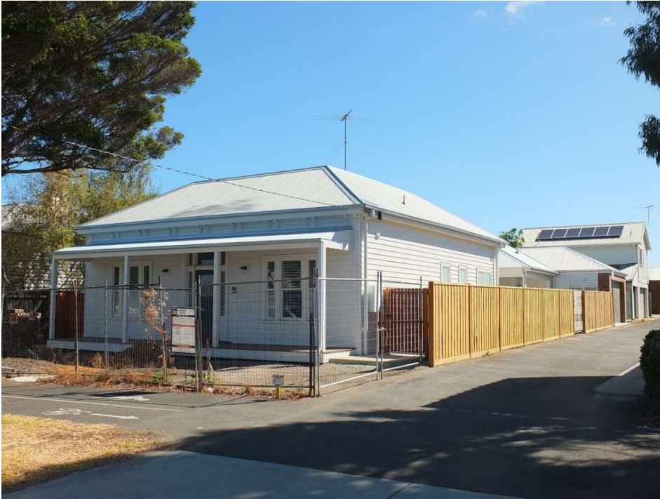
Lara Villa, almost completed (the new front fence yet to be constructed), 2024. Source: David Rowe.
