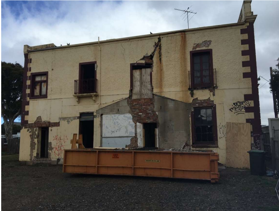
245 Malop Street, rear (north) elevation, August 2021. Source: Jennifer Bantow.
