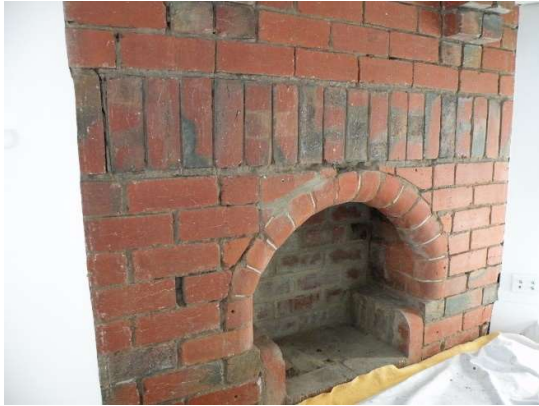
Fireplace, Geelong West, prior to restoration & tuckpointing. Source: Nat De-Palma.
