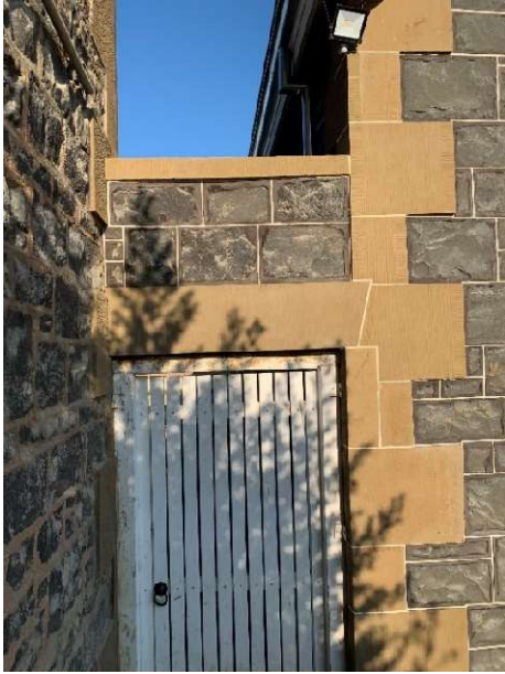
Gateway following restoration, 2023. Source: Matt Cartlidge.
