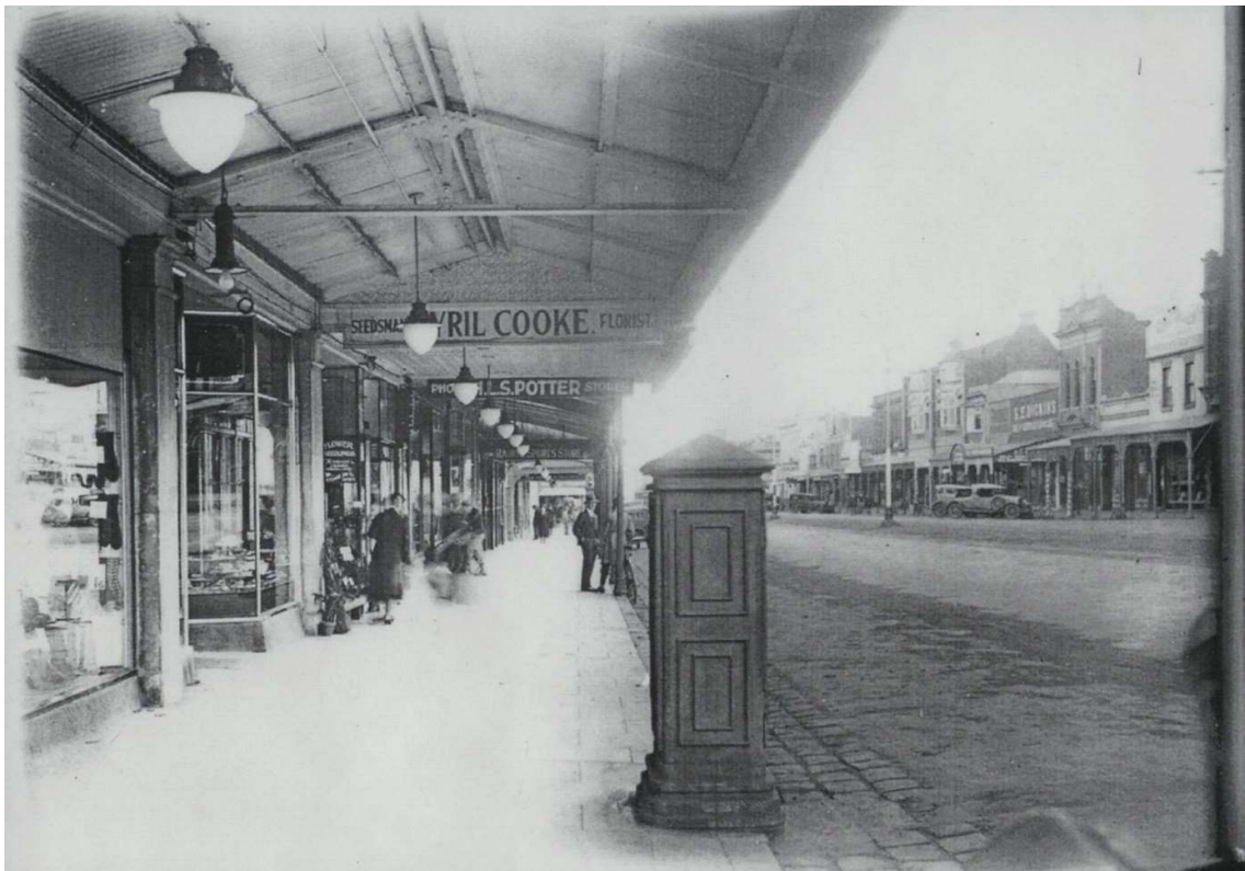
Underside of the cantilevered verandah, Ryrie Street, looking east, c.1912. Source: Kevin Krastins.
