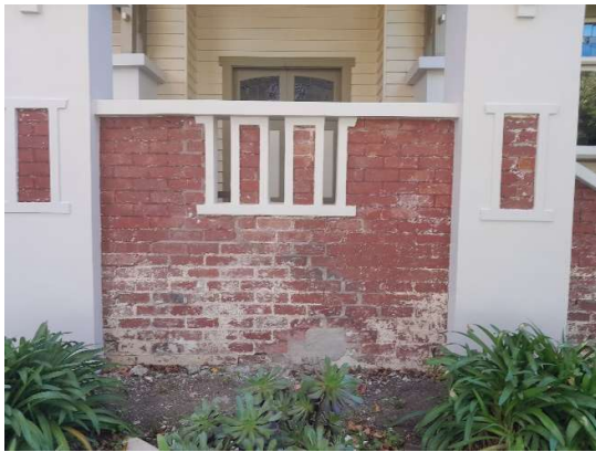
Verandah balustrade, Geelong, prior to restoration & tuckpointing. Source: Nat De-Palma.
