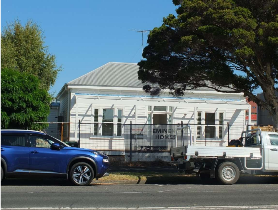
Lara Villa showing work in progress, including the new windows and front verandah under construction, 2024. Source: David Rowe.
