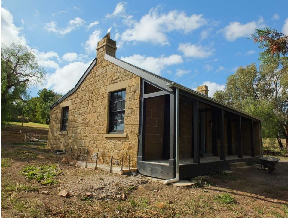
'Barwonside', 2024. Source: David Rowe.
