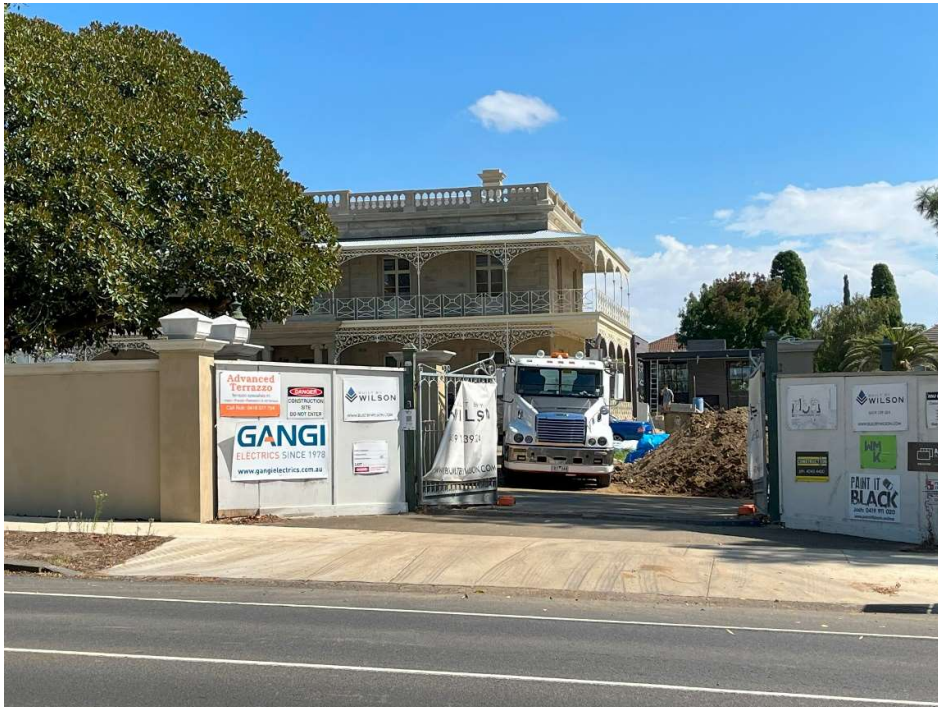
Works in progress, 28 March 2022. Source: David Rowe.
