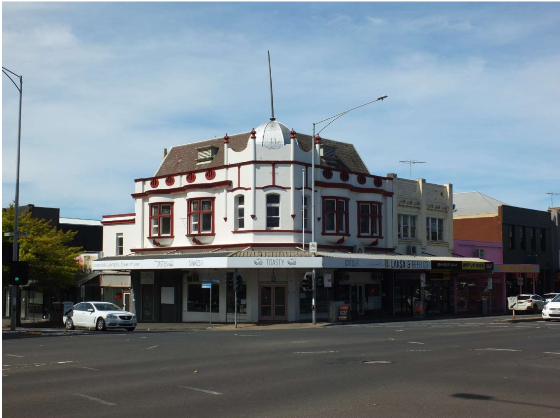
Former Macrow's Furniture Arcade, 15 February 2024. Source: David Rowe.
