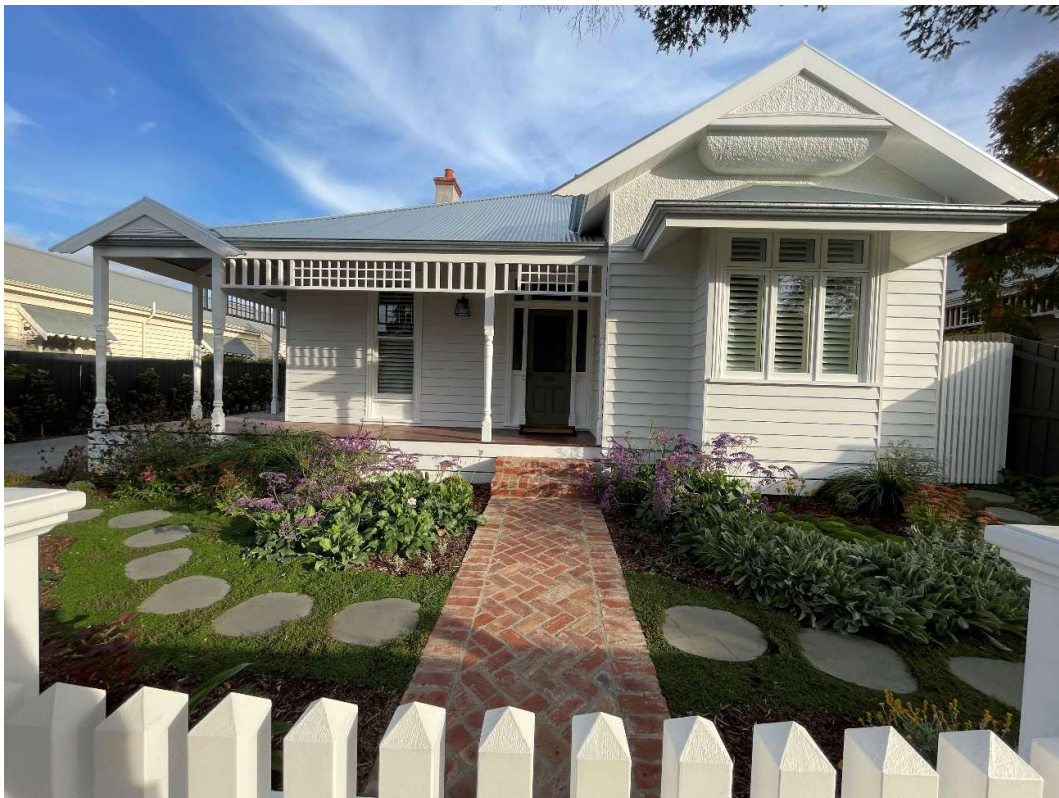
7 Lawton Avenue, almost complete, 2024. Source: Lauren Di Mauro
