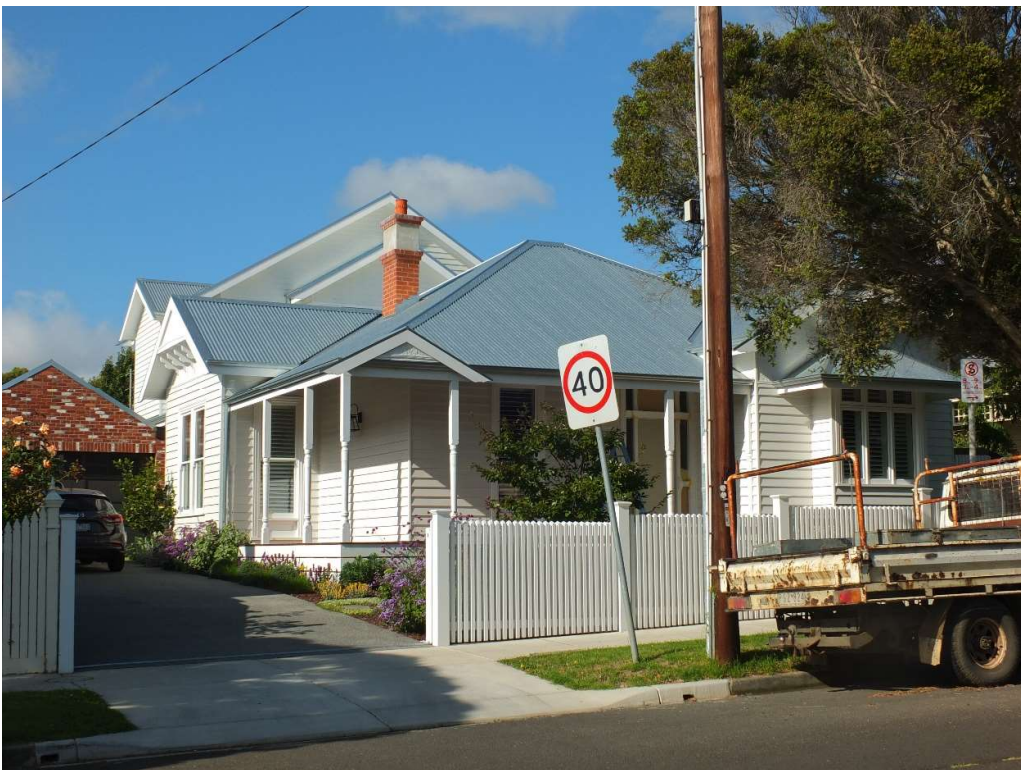
Dwelling, 7 Lawston Avenue, with restoration in progress, 2024. Source: David Rowe.
