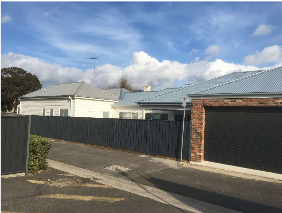
Rear additions and garage as viewed from the lane, 2024. Source: Jennifer Bantow.
