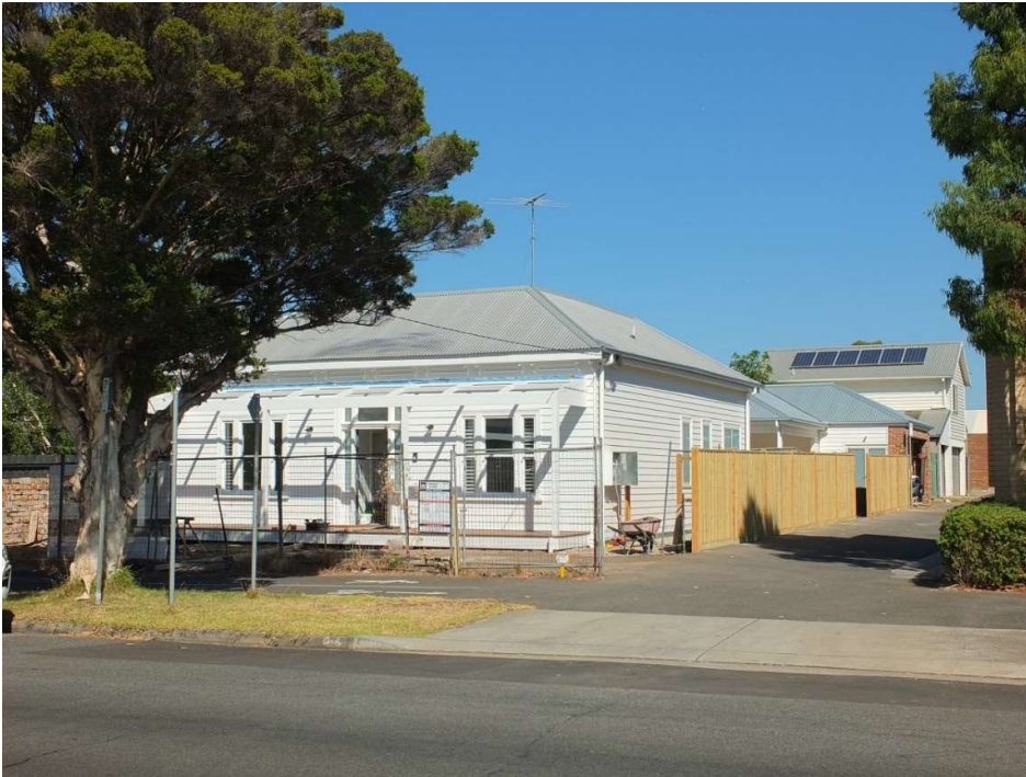
Lara Villa showing work in progress, including the new windows and front verandah under construction, as well as the rear additions, 2024. Source: David Rowe.
