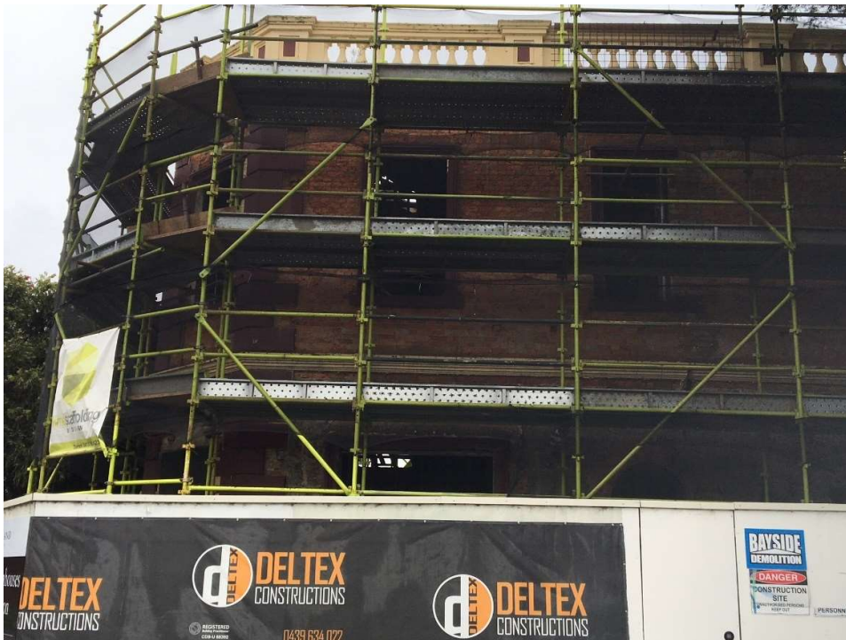
245 Malop Street, showing early rendered removed, and wall repairs being carried out prior to re-rendering and painting, October 2021. Source: Jennifer Bantow.
