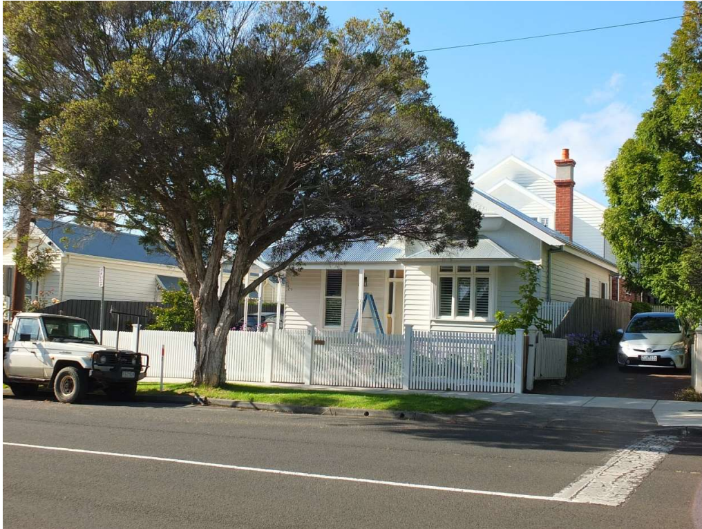
Dwelling, 7 Lawton Avenue, with restoration in progress, 2024. Source: David Rowe.
