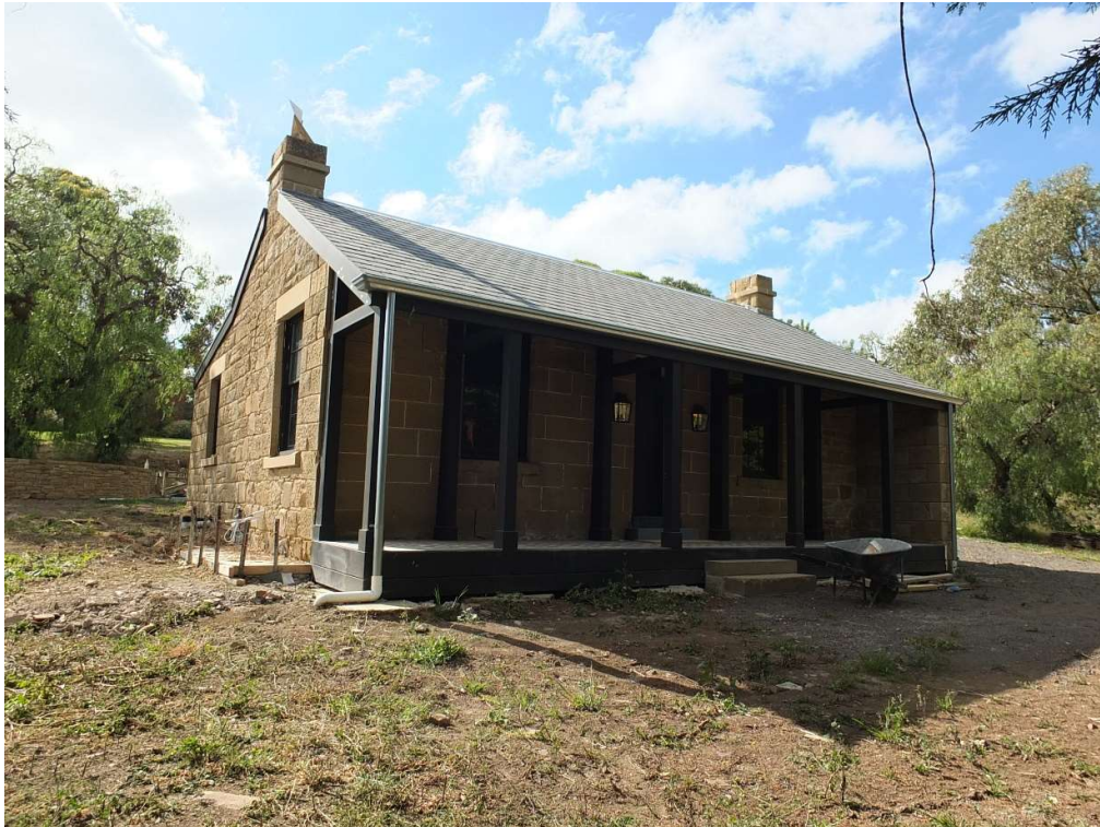
'Barwonside', 2024. Source: David Rowe.
