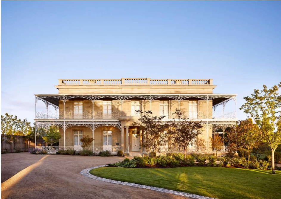
Armytage House restored and partially reconstructed, 2024. Source: Novka Long, Indre Design.
