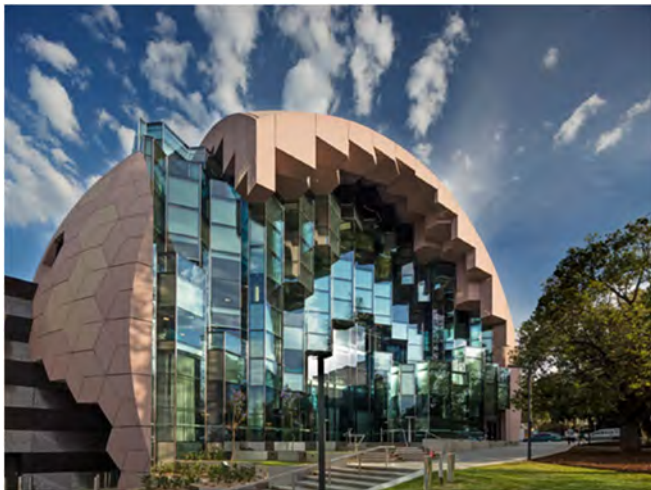
THE GEELONG LIBRARY AND HERITAGE CENTRE SHOWCASES SUSTAINABILITY IN THE BUILT ENVIRONMENT WITH ITS 5 STAR GREEN STAR RATING
