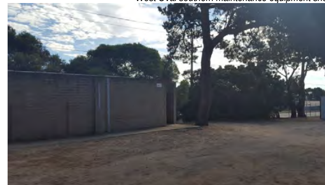
West Oval northern toilets
