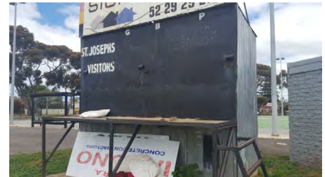
NH Drew Oval – Redundant Manual AFL scoreboard
