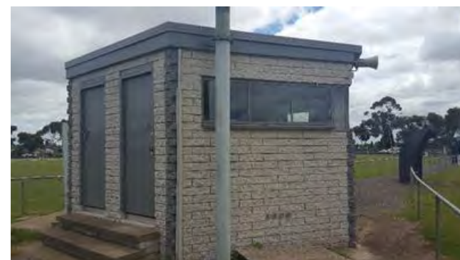
Existing Time Keepers Box / Storage Shed
