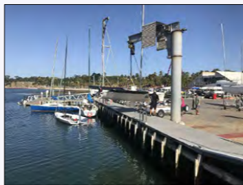
VESSEL LAUNCHING / RETRIEVAL CRANE
