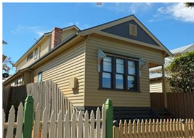
Completed works, including substantial repairs, rear additions and chimney reconstruction. Source: Dr David Rowe.
