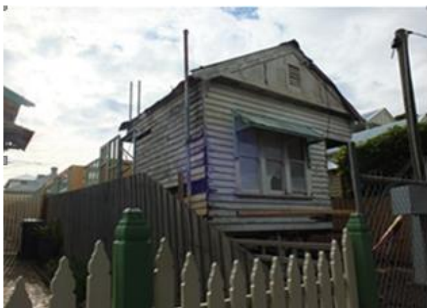
Dwelling temporarily propped during demolition and construction. Source: Dr David Rowe.
