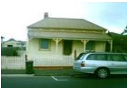
Before Repair. Source: Dr David Rowe.
