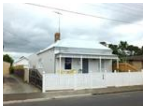
After Repair. Source: Dr David Rowe.
