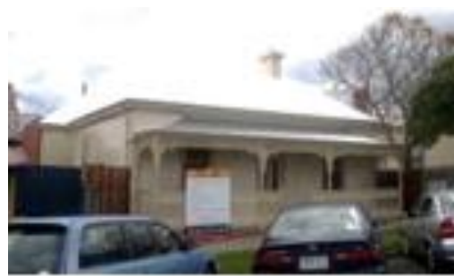
After Repair. Source: Dr David Rowe.
