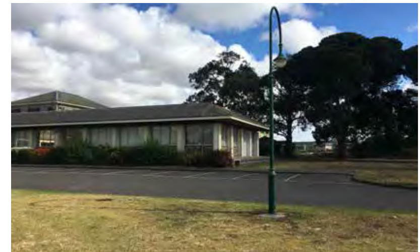
Eastern wing of 1960s Corio Shire extension
