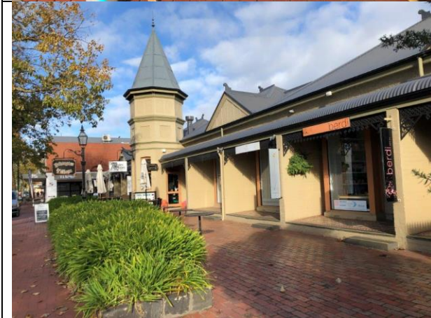
General view. All these retail units have a stepped entry and are stepped back from main footpath.
