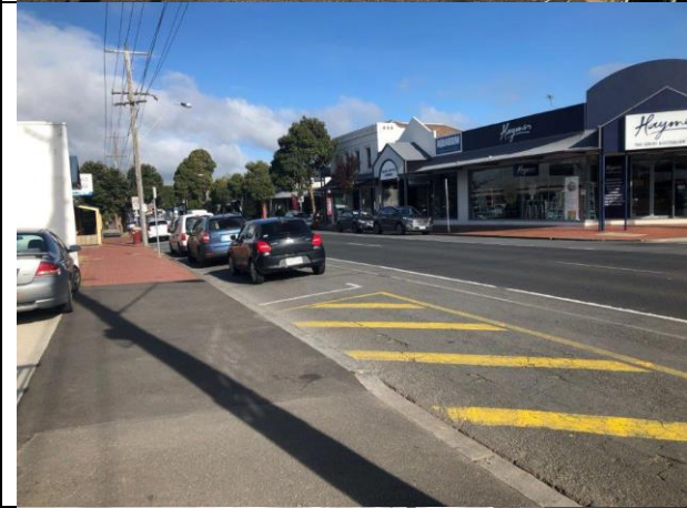
View north. Asphalt footpath, asphalt crossovers; abutment with brick footpath.
