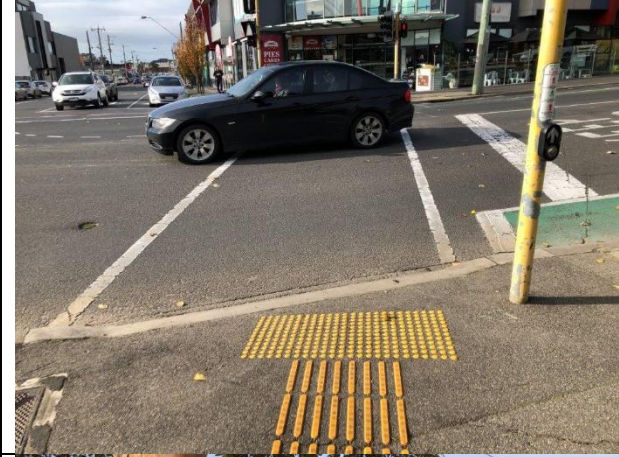
Controlled crossing across Pakington Street, footpath grades down to carriageway with gradient approx. 8.7%
