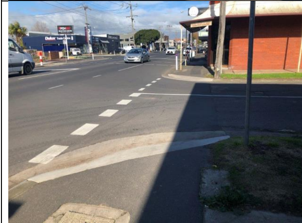
Crossing across Clonard Avenue, footpath grades down to carriageway with gradient approx. 14.3%
