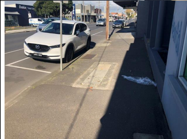
General view – multiple repairs adjacent utility covers
