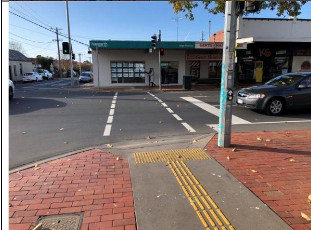
Controlled crossing across Pakington Street, footpath grades to carriageway with gradient approx. 9.6%
