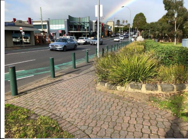
General view Footpath slope approx 7.0% (1:14) towards road. Consider additional barrier adjacent road.
