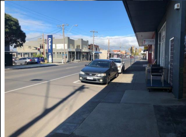
General view – multiple repairs
