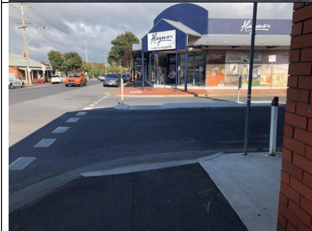
Crossing across Isabella Street, footpath grades to carriageway, gradient approx. 19.8%
