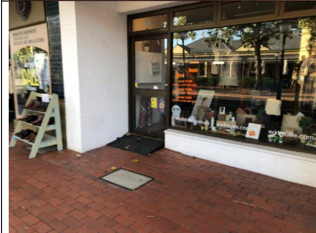
Example showing footpath and retail entrance with temporary ramp.
