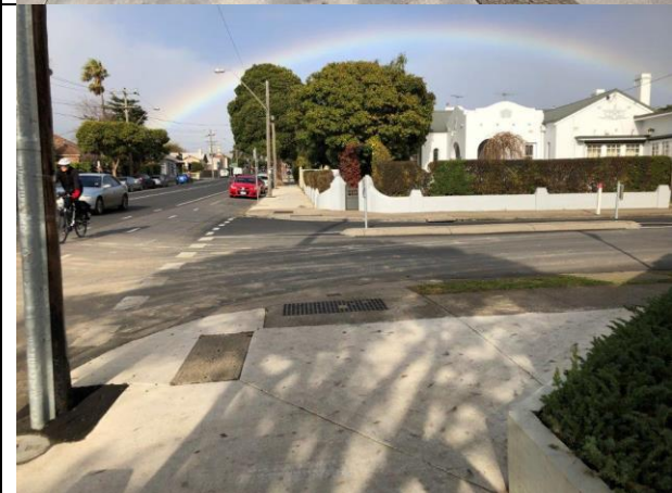
Crossing across Gertrude Street, footpath grades down to carriageway with gradient approx. 0.2% × Kerb cut not aligned with path of travel
