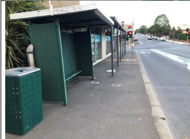
× Bus shelter located at distance to bus stop × Awning poles constrict free movement between bus shelter and bus stop.
