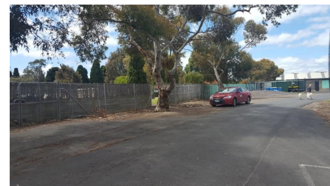
Sealed roadway to north of Walker Oval
