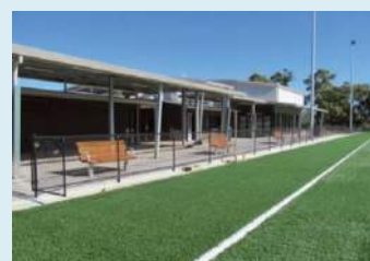
Monbulk Soccer Centre (by Devco Construction for Yarra Ranges Council)
