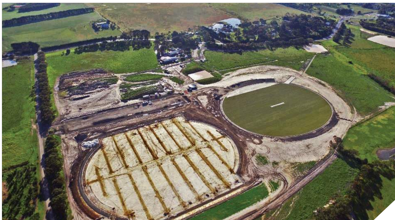
Image above: Aerial photo of Stage one construction works for the Drysdale Sporting Precinct in September 2017 (image credit: Drysdale Sporting Precinct Funding Now)
