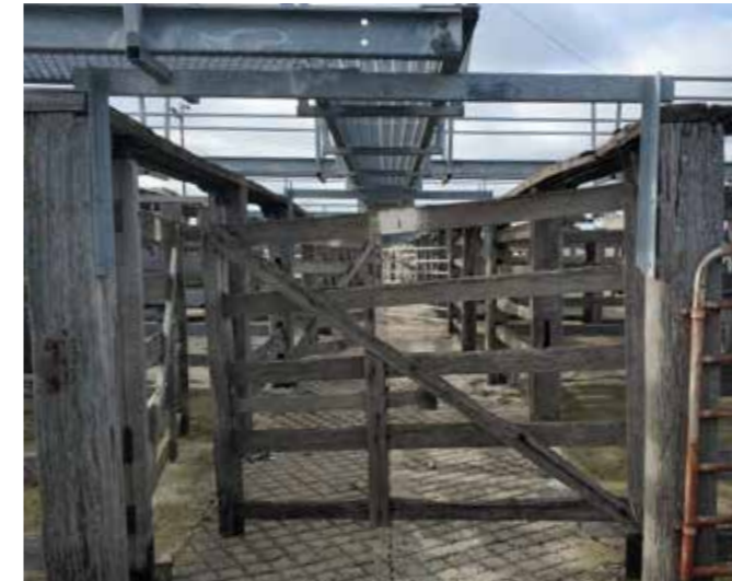
3 First rows for cattle yards to be retained as shown on the plan.
