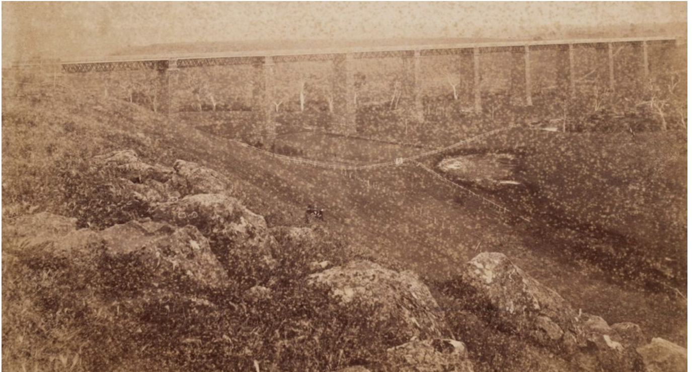
Figure 1.17: C. Nettleton, Moorabool Viaduct showing cliff faces, c.1875. Source: accession H84.79/1, State Library of Victoria.
