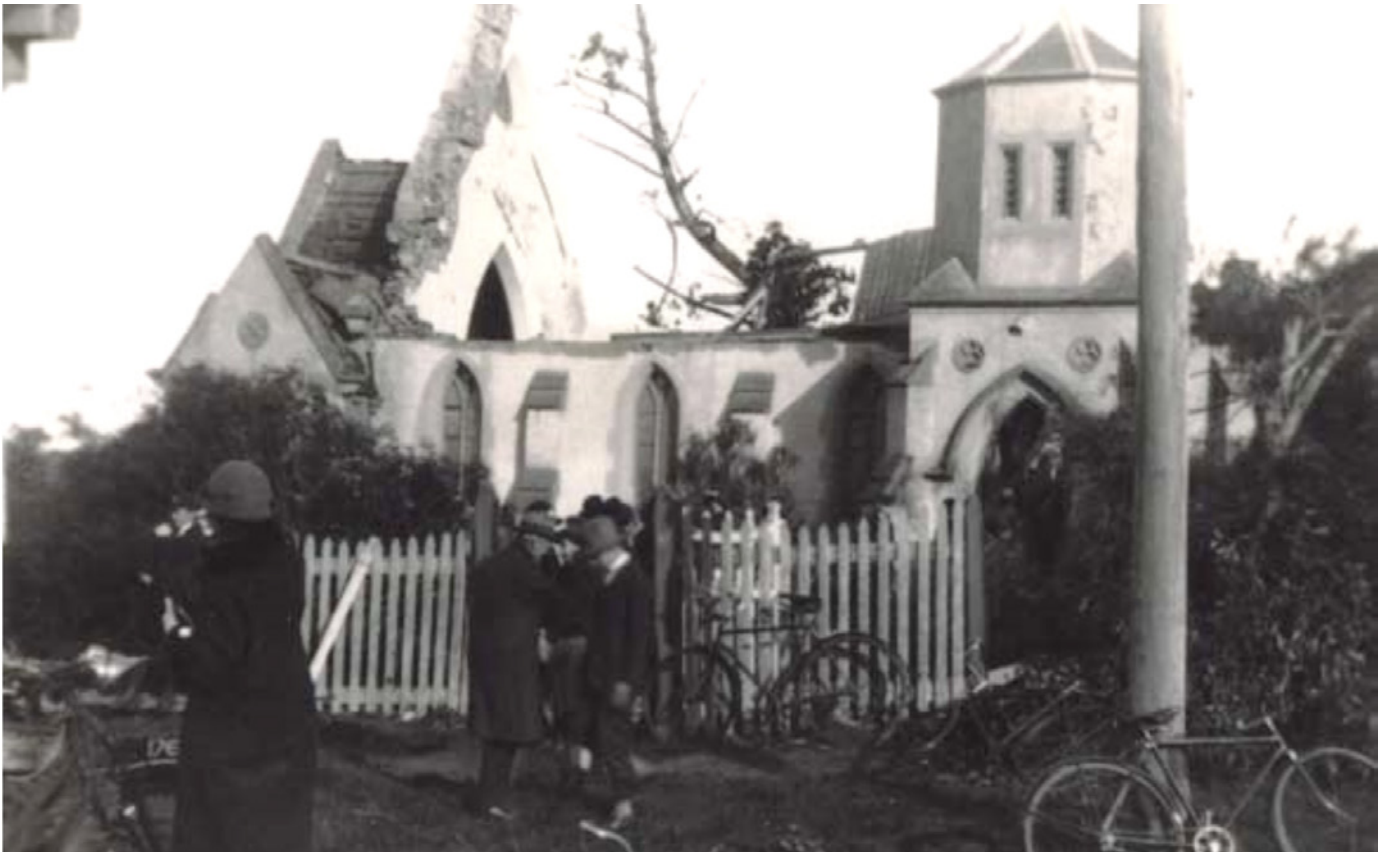
Figure 1.33: Substantially damaged St. John's Anglican Church, Highton, following tornado, 1926. Source: GRS 2009/04670, Geelong Heritage Centre collection.
