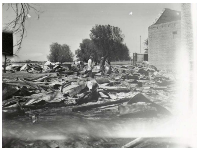
Figure 1.29: K. Felloes, Two girls wander among the ruins of their school library at Lara East, which was destroyed in the bushfire, Australian News & Information Bureau, 1969. Source: Bib ID 4589309, National Library of Australia.
