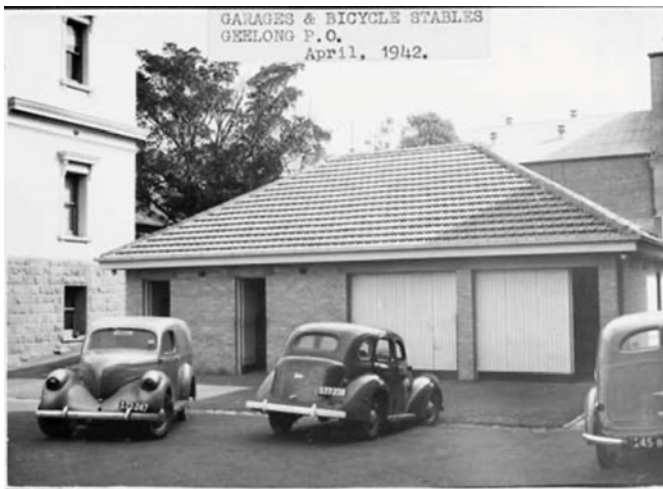
Figure 3.58: Geelong Post Office, 'Garages and Bicycle Stables', April 1942 (now demolished). Source: NAA: B5919.13/227, National Archives of Australia.
