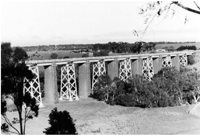
Figure 3.105: Moorabool Viaduct, 1998. Source: David Rowe.
