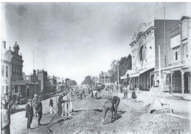
Figure 3.85: Ryrie St (between Moorabool & Yarra Streets), with tram line under construction, c.1922. Source: McDonald collection, Kevin Krastins, City of Greater Geelong.
