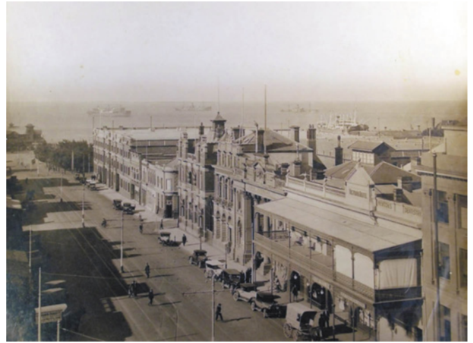
Figure 3.79: Moorabool St, looking north-east, showing cast iron & timber electricity poles for tram service at the centre & sides of the street, c.1930. Source: GRS 2009/1304a, Geelong Heritage Centre collection.
