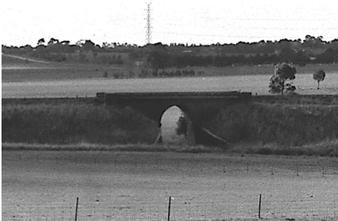
Figure 3.102: Railway bridge, Moorabool, 1998. Source: David Rowe.
