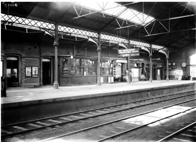
Figure 3.119: Geelong Railway Station Train Hall & Platform 1, photographic collection, railway negatives, c.1920s. Source: VPRS 12903/P1, it 261/05, Public Record Office Victoria.
