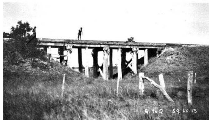
Figure 3.109: Railway Bridge, Geelong to Queenscliff line, photographic collection, railway negatives, 1885. Source: VPRS 12800/P1, H 4666, Public Record Office Victoria.
