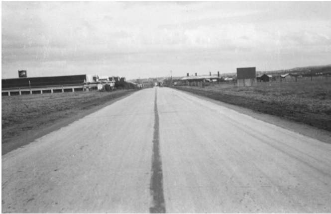
Figure 3.09: Concrete section, Geelong to Melbourne Road, North Geelong (note the Ford Motor Company on the left in the background), photographic collection, Roads Corporation, 1929. Source: VPRS 17684/P3 it 28/00087, Public Record Office Victoria.
