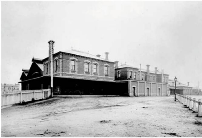
Figure 3.118: Geelong Railway Station, east and south elevations, photographic collection, railway negatives, c.1900. Source: VPRS 12800/P1, Unit 195 Public Record Office Victoria.
