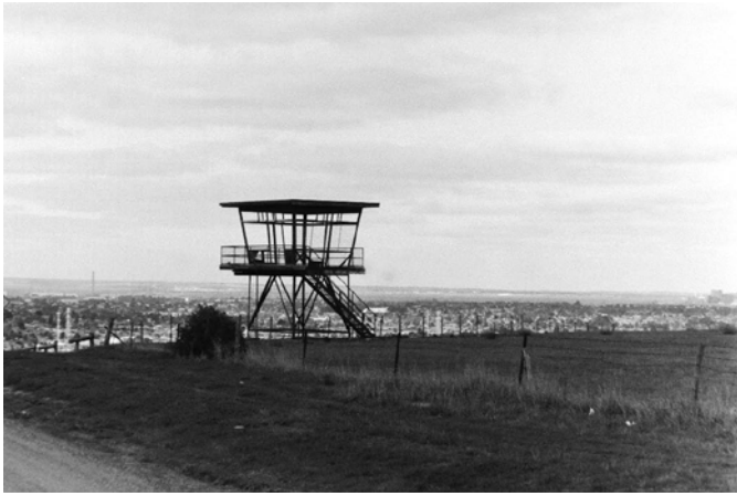
Figure 3.177: Abandoned air traffic control tower, Lovely Banks airport, 1999. Source: David Rowe.
