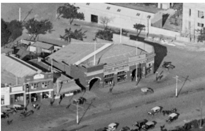
Figure 3.67: C. Pratt, Balfours' Garage, Mercer Street, c.1925 (right). Also note Richardson's two storey garage (original wing) on the left. Source: accession H91.160/838 State Library of Victoria.
