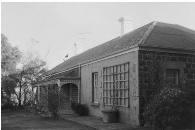
Figure 3.103: 'Craigton', original residence of Mr Duxbury, Moorabool, 1998. Source: David Rowe.
