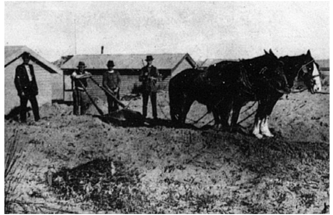
Figure 3.16: Road making at Barwon Heads by returned soldiers, 1919. Source: News of the Week , 11 September 1919, GRS 2121, Geelong Heritage Centre collection.
