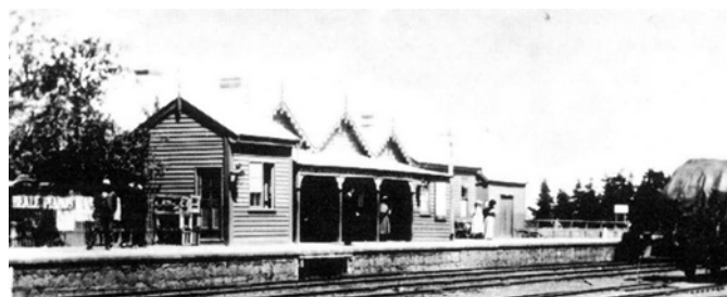
Figure 3.123: Lara Railway Station, n.d. [c.1900]. Source: K. Eastman in From Duck Ponds to Lara , p.60.
