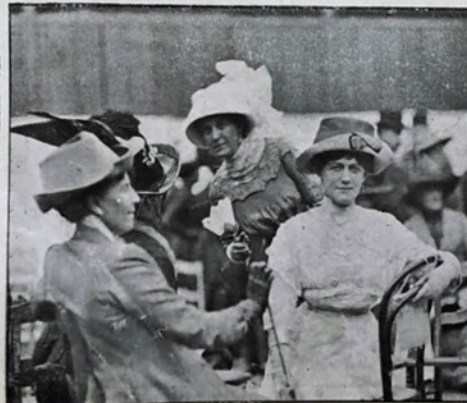
AT THE POWER HOUSE
