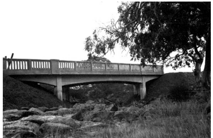
Figure 3.37: Newly completed Ripley Bridge, photographic collection, Roads Corporation, 1928. Source: VPRS 17684/P3 it 28/00022. Public Record Office Victoria.
