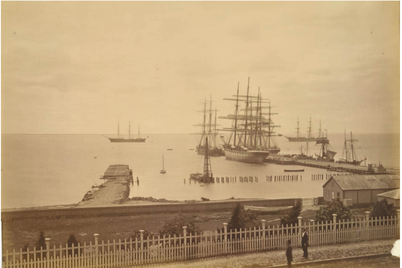
Figure 3.140: F. Kruger, Yarra Street, wharves, Geelong (the ruinous former Steampacket Wharf is shown on the left, with remnant piles extending to Yarra Street Wharf on the right), c.1878. Source: accession PH208-1979, National Gallery of Victoria, Melbourne. Gift of Mrs Beryl M. Curl, 1979.
