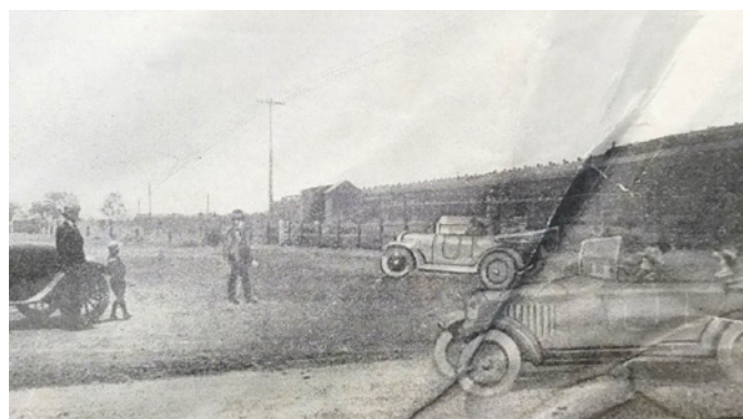
Figure 3.122: North Shore Railway Station (background), c.1926. Source: Bay View Estate Plan, n.d., Special Collections, Deakin University Library.
