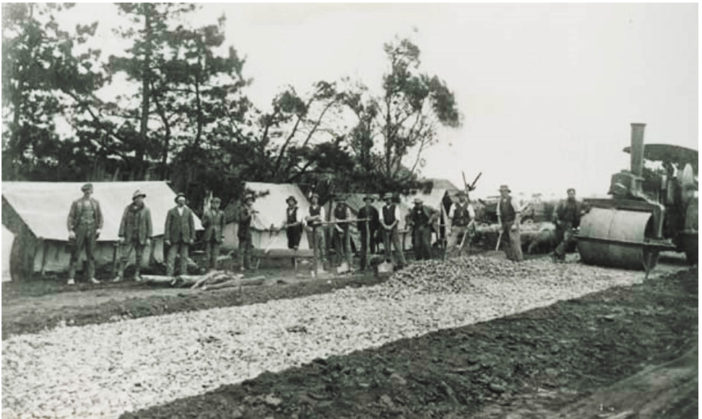
Figure 3.17: Road making, Torquay Road, c.1917-18. Source: GRS 2009/01846/062 Geelong Heritage Centre collection.
