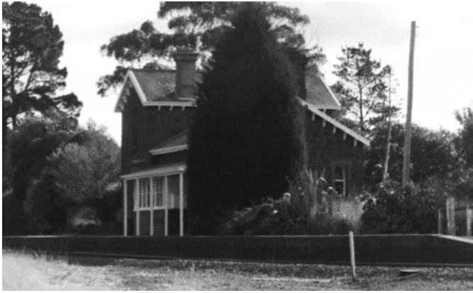
Figure 3.128: Moorabool Railway Station, 1998. Source: David Rowe.
