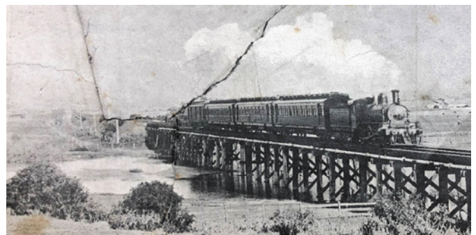
Figure 3.107: Breakwater Rail Bridge, 1911. Source: News of the Week , 6 July 1911, GRS 2121/3, Geelong Heritage Centre collection.
