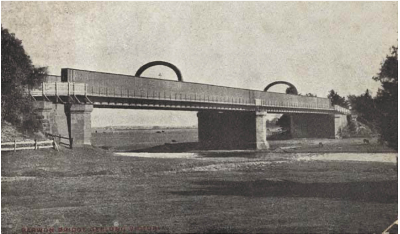
Figure 3.22: Barwon Bridge, c.1910. Source: GRS 6996/0 Geelong Heritage Centre collection.
