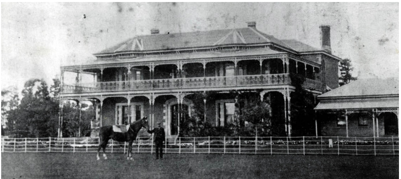
Figure 4.04: Pirra Homestead, c.1910. Source: GRS 2009/01847/134, Geelong Heritage Centre collection.
