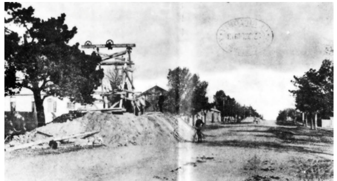
Figure 4.128: Sewerage shaft, Bellerine Street (near Myers Street), 1913. Source: News of the Week , 19 June 1913, GRS 2121, Geelong Heritage Centre collection.
