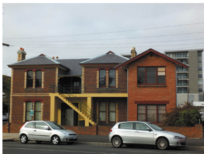
Figure 4.101: 'Waverley', 94 Western Beach Road, 2014. The original wing is on the left, the addition of 1873 (centre). Source: David Rowe.
