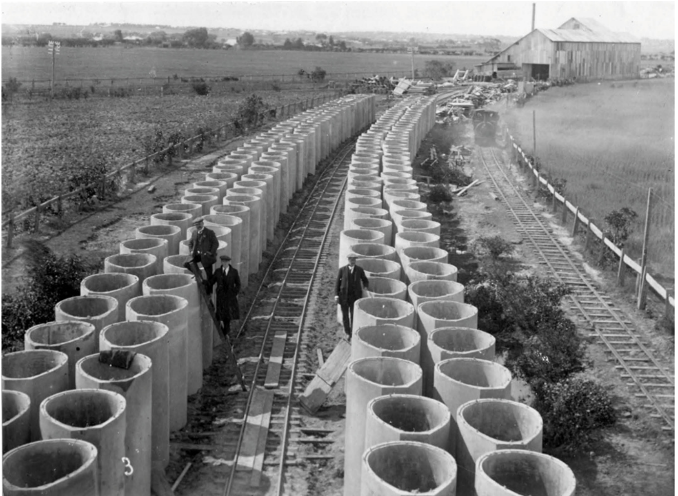
Figure 4.127: Curing yard for ovoid concrete pipes, Marshall, c.1912. Source: Barwon Water.
