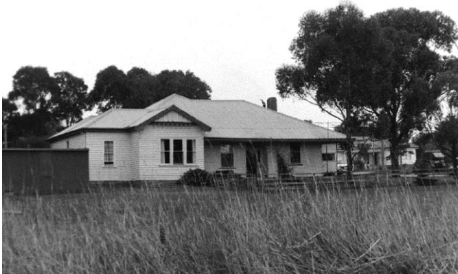
Figure 4.46: 'Sparrovale' Manager's House, 1998. Source: David Rowe.
