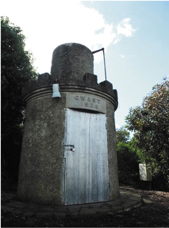
Figure 4.121: Former valve tower to the Bell Post Hill basin, Heritage Drive, Hamlyn Heights, 2019. Source: David Rowe.
