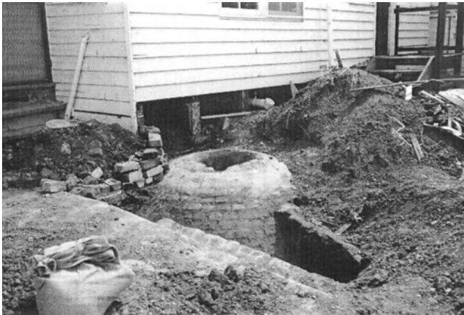
Figure 4.113: Excavations exposing underground tank at rear of 1 Little Ryrie St, Geelong, 1998. Source: David Rowe.
