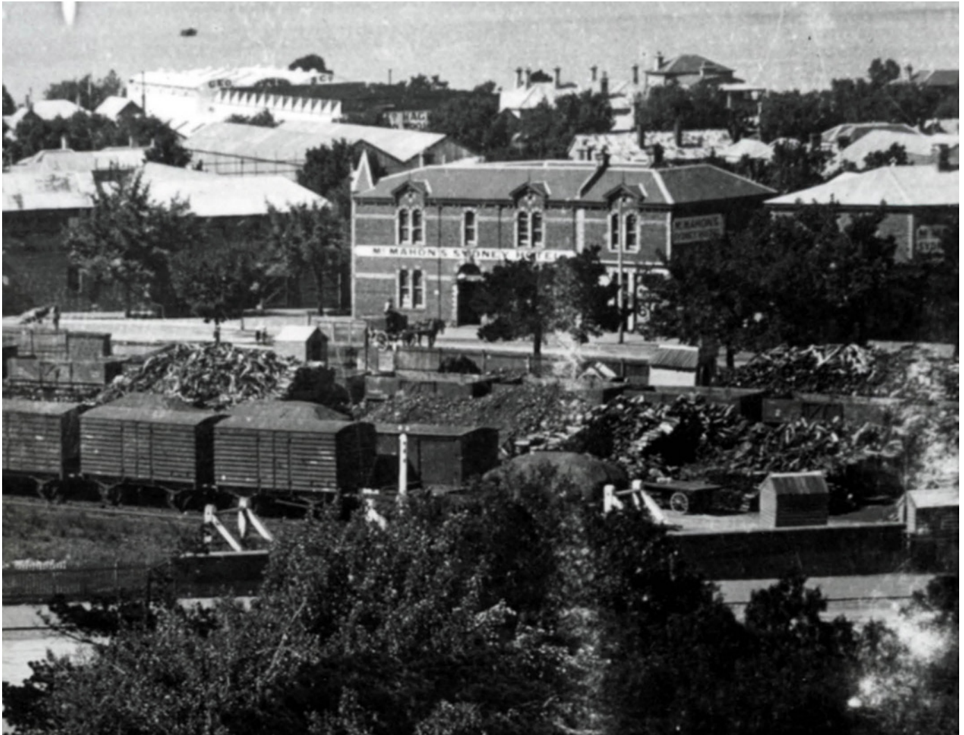
Figure 4.98: McMahon's Sydney Hotel, Mercer Street, Geelong, 1910, where Widdicombe's brick were used for the first time in 1872. Source: GRS 2009/01703/111, Geelong Heritage Centre collection.
