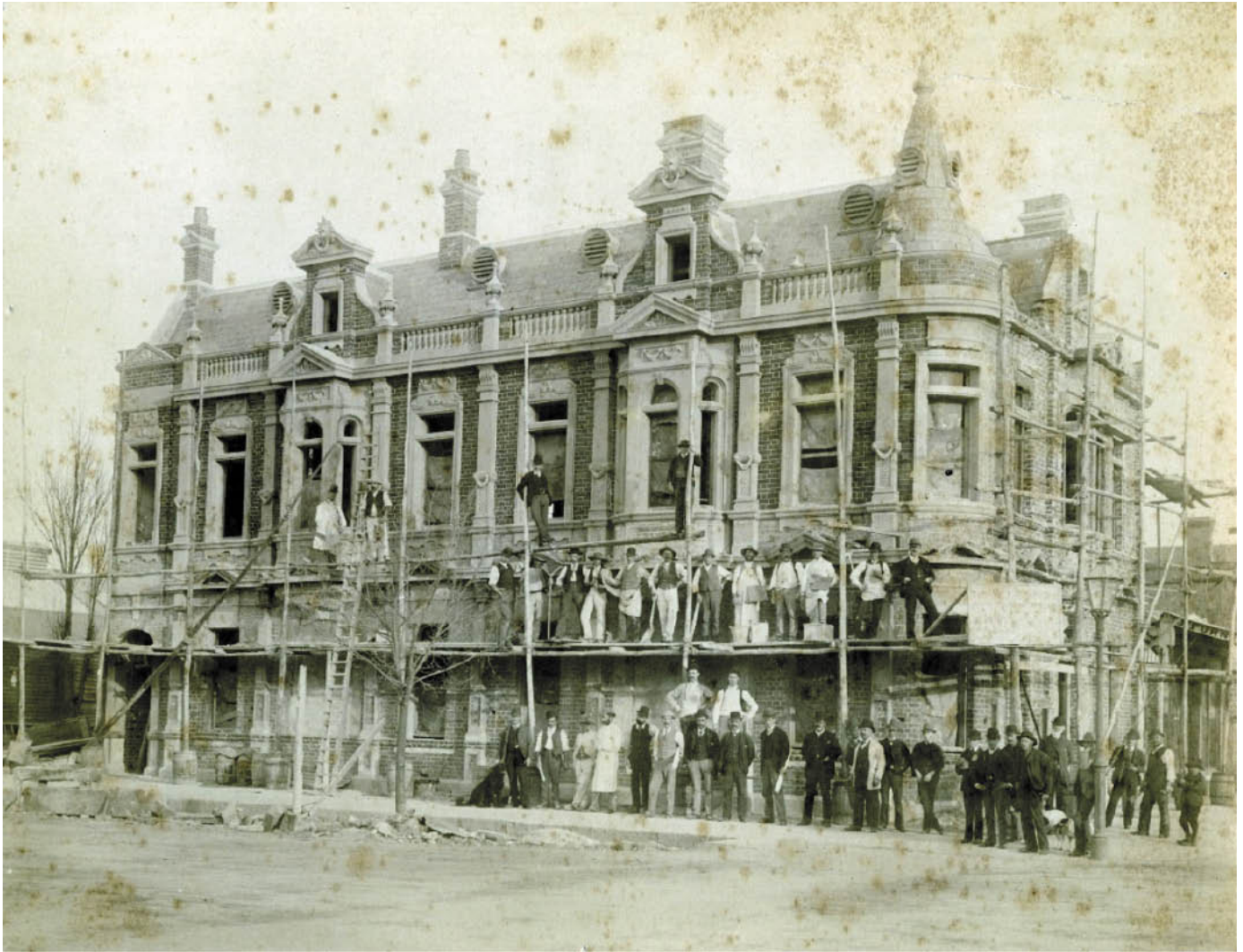
Figure 5.180: Corio Chambers building nearing completion, 33 Yarra Street, Geelong, 1890. Source: GRS 2009/03681, Geelong Heritage Centre collection.
