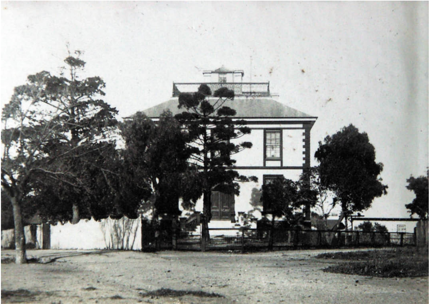
Figure 5.34: T.T. Holmes, 'Fairfield Hall', corner Myers Street & Bourke Crescent, c.1931 (now demolished). Source: Holmes collection, Authentic Heritage Services.
