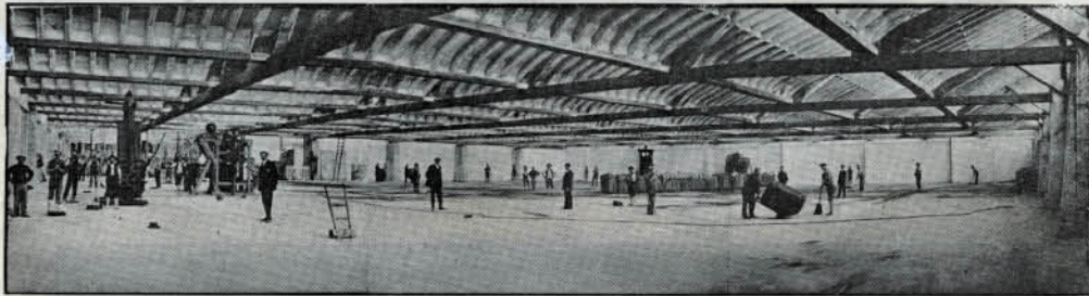
NEW SHOW FLOOR CLEAR OF TEMPORARY SUPPORTS.
