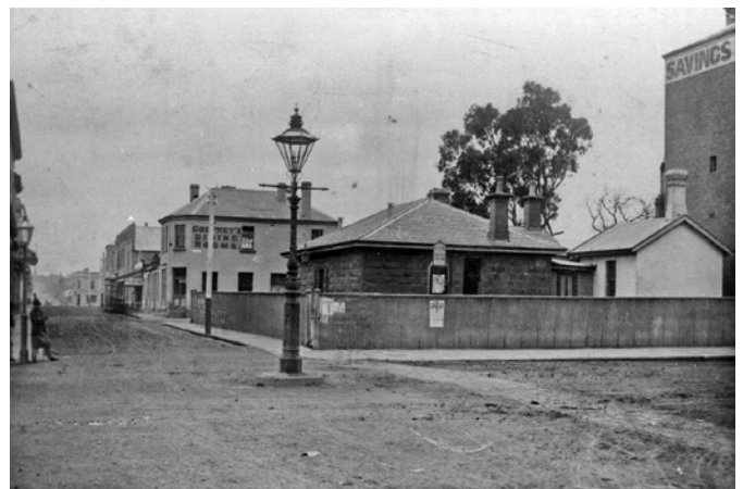
Figure 7.44: Watch House/Police Station, corner Moorabool & Corio Street, n.d. [c.1900]. Source: Wynd collection, image p64r03f04, Authentic Heritage Services Pty Ltd.
