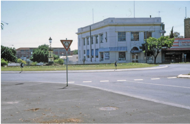
Figure 7.95: Round-about, corner Gheringhap & Malop Streets (removed early 21st century), 1995. Source: Wynd Collection, Authentic Heritage Services.
