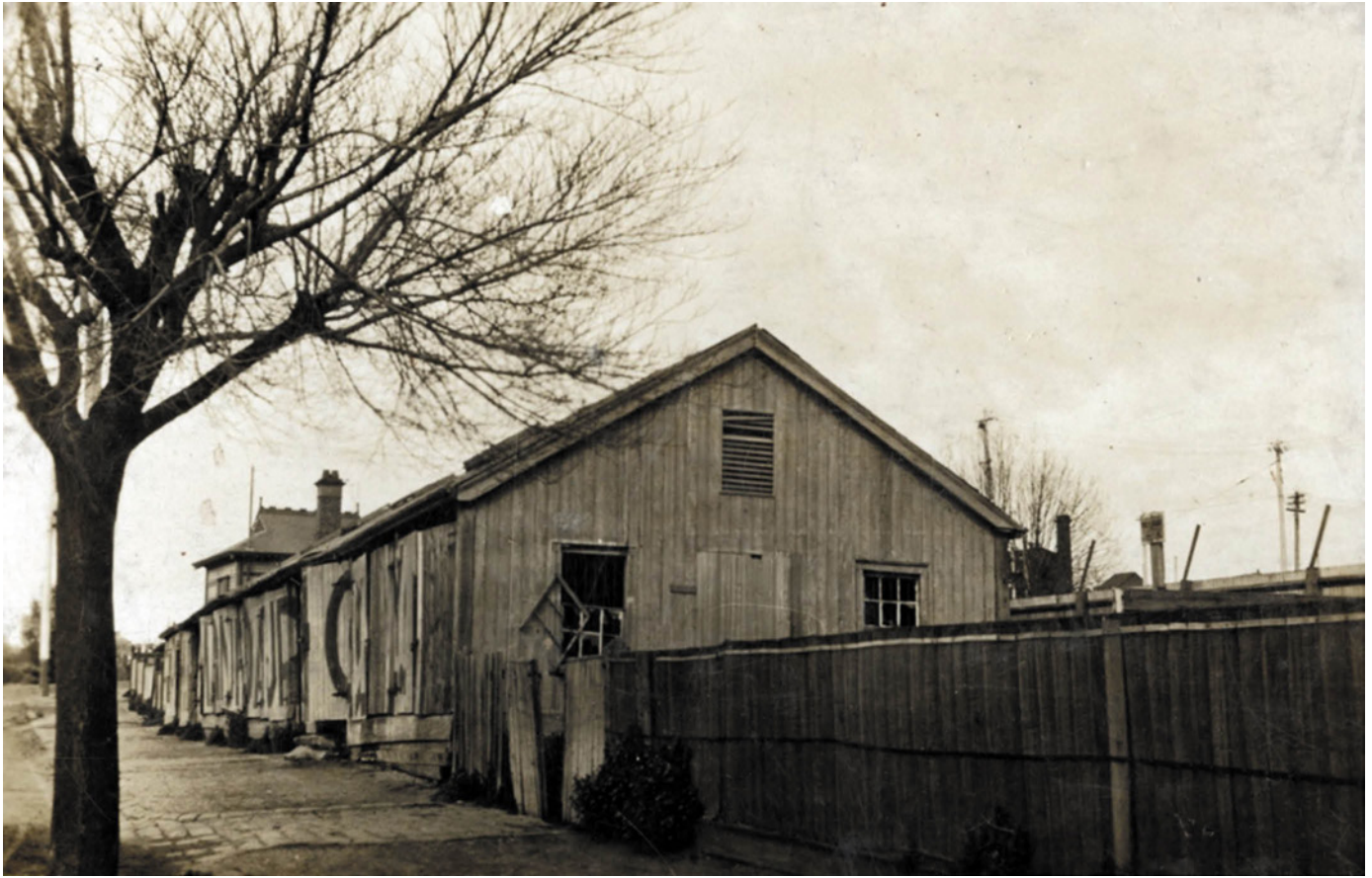
Figure 7.66: Customs Gauging Shed, corner Moorabool Street & Eastern Beach Road, c.1920. Source: GRS 2009/00280 Geelong Heritage Centre collection.
