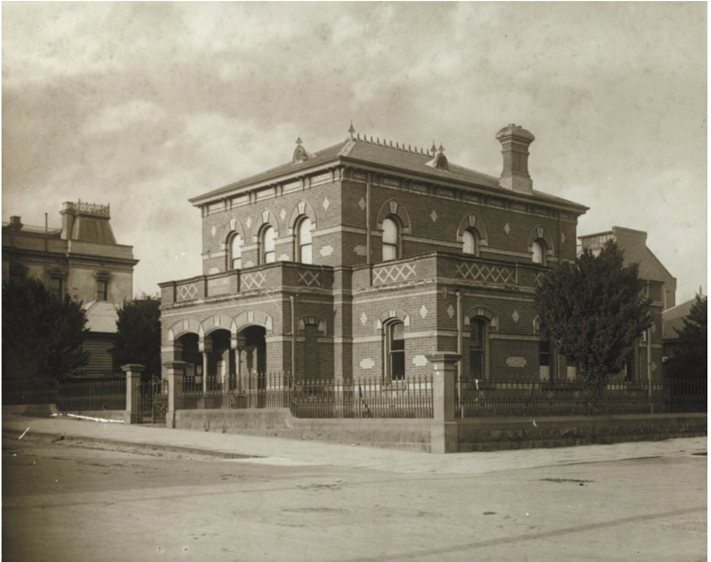
Figure 7.51: Geelong Police Court House, Gheringhap Street, c.1915. Source: GRS 2009/01311, Geelong Heritage Centre collection.
