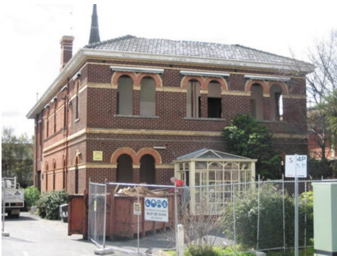
Figure 7.89: Former Country Roads Board Building (Police Station), at time of demolition, August 2008. Source: Jennifer Bantow, Geelong.
