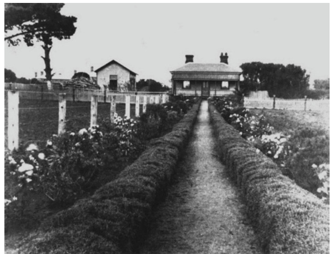
Figure 7.55: Drysdale Police Residence (centre) and station (left), n.d. Source: Image 0335, Bellarine Historical Society.
