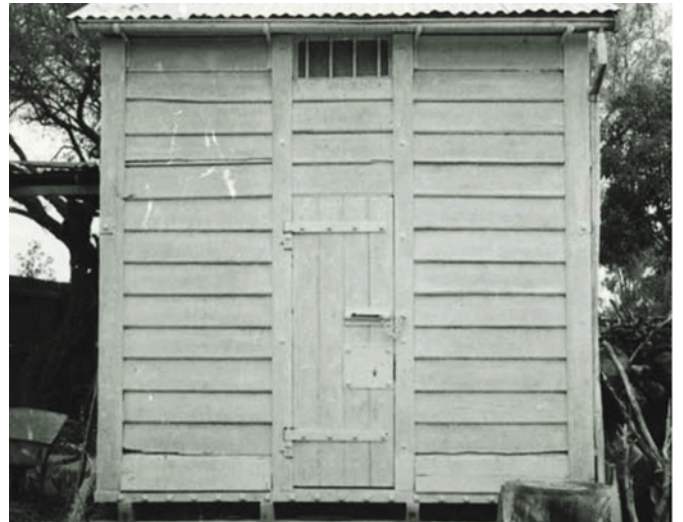
Figure 7.61: Lock Up, Drysdale, 27 November 1956. Source: GRS 2020/12 Geelong Heritage Centre collection.
