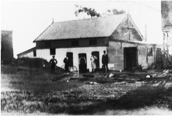
Figure 7.76: Former Drill Hall (Bellarine Dairy Co. Butter Factory), c.1930s. Source: Bellarine Historical Society image s24m29, Bellarine Historical Society.
