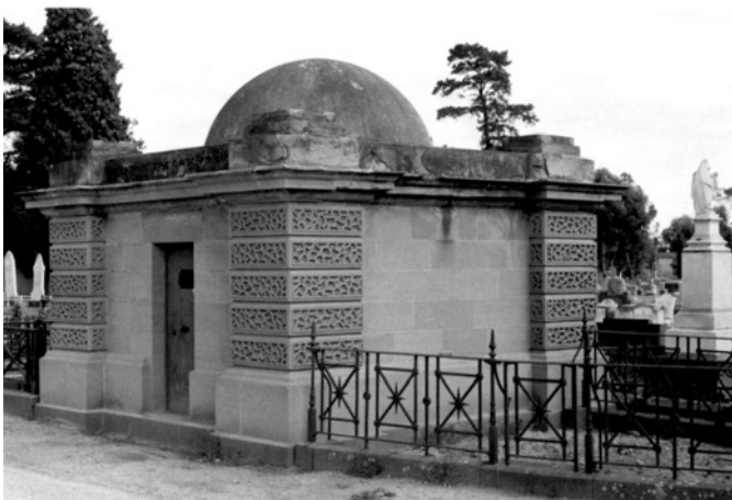
Figure 8.177: J.T. Collins, Strachan family mausoleum, Western Cemetery, 27 April 1978. Source: accession H63.210/356, State Library of Victoria.
