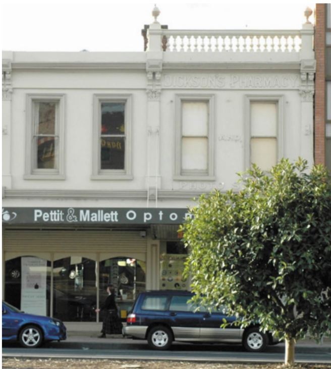
Figure 8.125: Former Dickson's Pharmacy building (right), 121 Ryrie Street, 2005. Source: David Rowe.
