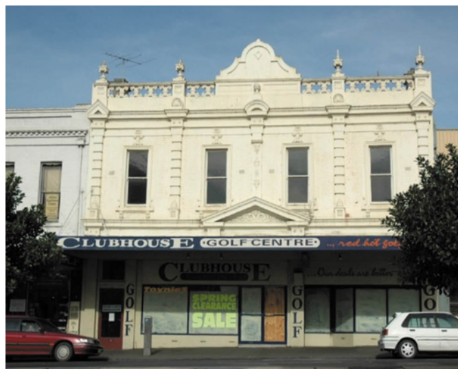
Figure 8.150: Former YMCA Building, 72-76 Ryrie Street, 2005. Source: David Rowe.
