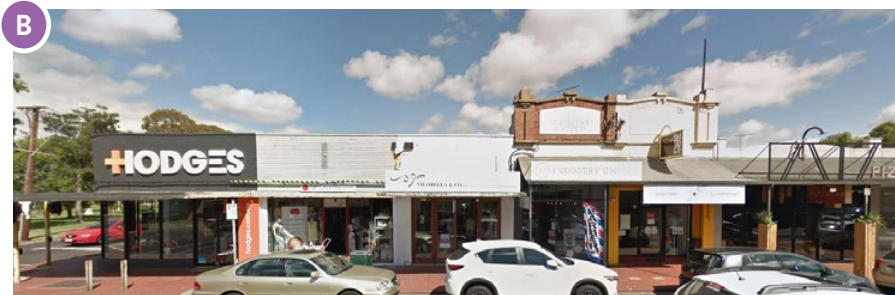
Shop frontages along Pakington Street between Autumn and Yuille Streets.
