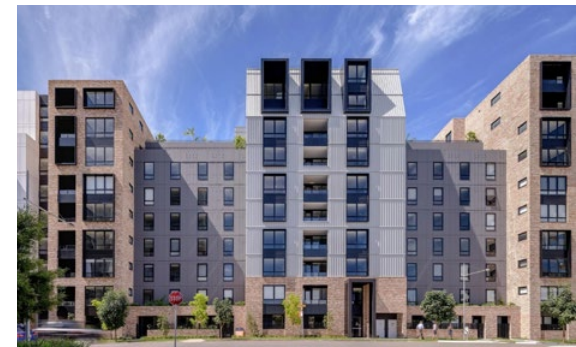
Lumina Apartments, DKO
