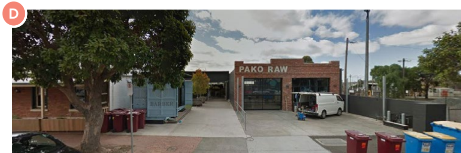
Examples of buildings with entrances set back from Pakington Street.
