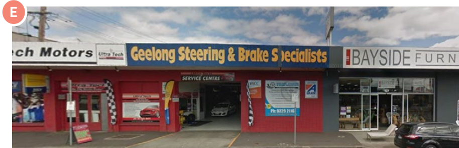
Examples of buildings along Pakington Street with larger grain and wide frontages.
