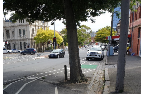
(b) Northbound bicycle lane diversion around tree
