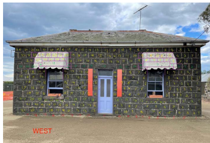
Demolition and conservation images
