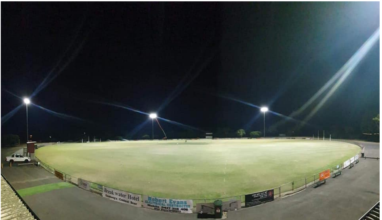
New sports lighting on Oval 1 at Grinter Reserve (completed February 2021)
