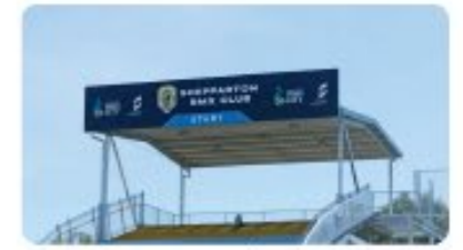
Shade structure to BMX starting hill
