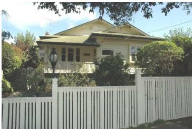
Fig. 22: Fence stepped along slope of boundary. Source: Dr David Rowe.
