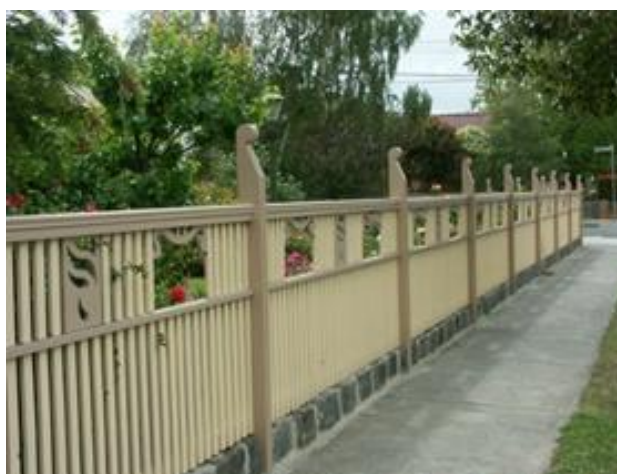
Fig. 8: Detail of Federation era picket fence with fretwork capping. Source: Dr David Rowe.
