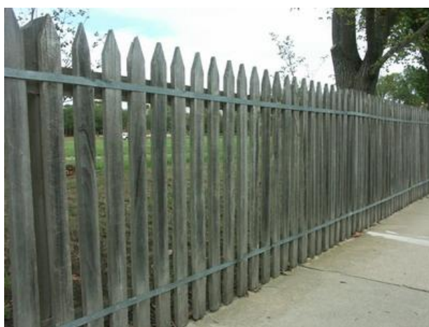
Fig. 3: Unpainted timber picket fence with hoop iron used to reinforce the pickets. Source: Dr David Rowe.
