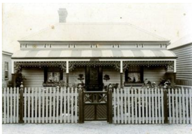
Fig.1: Victorian dwelling with pointed timber picket fence, expressed posts with decorative cappings, and timber gate. Source: Emerald Museum.
