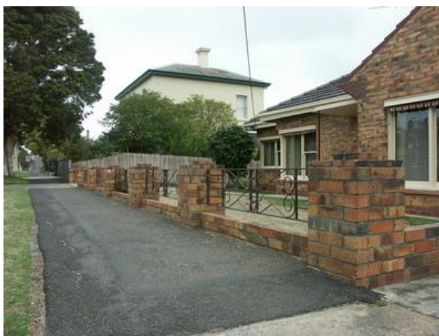
Fig. 19: Low brick fence with open bays with trussed geometric panels. Source: Dr David Rowe.
