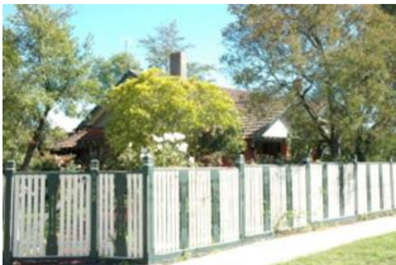
Fig. 14: Capped timber picket fence to an interwar Bungalow styled dwelling. Source: Dr David Rowe.
