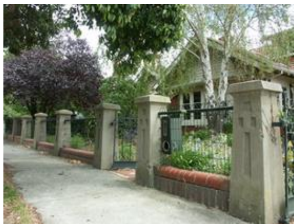
Fig. 12: More substantial woven wire fence to large property, with rendered piers and brick plinths. Source: Dr David Rowe.
