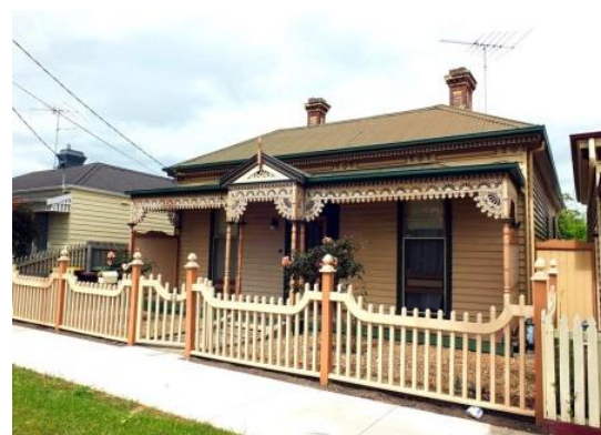
Fig 2: While the side (west) roof face locations of these panels are still visible to a street, the visual impact is less considerable than their placement on the front (north) roof face. Dr David Rowe.
