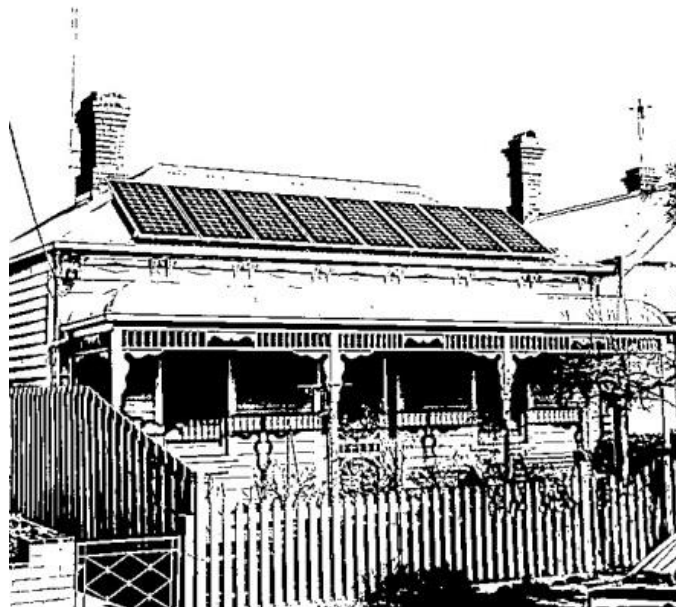
Fig 1: The installation of panels on the front roof face and projecting beyond the roof ridgelines of this Victorian dwelling has had a negative impact on its significance, character and appearance. Source: Dr David Rowe.
