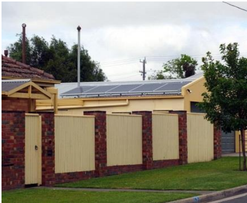
Fig. 3: The placement of solar panels on the north roof face of the rear garage - while still visible to a street - has greatly reduced the visual impacts compared to a location on the front roof of the dwelling where there was also potential to damage the roof tiles. Source: Dr David Rowe.
