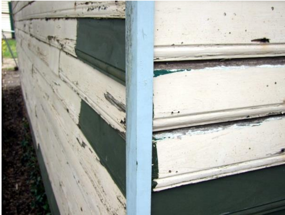
Detail of new weatherboards (dark colour) cut into existing weather wall cladding. The replacement material is therefore limited to where required only. Source: Brian Benson.
