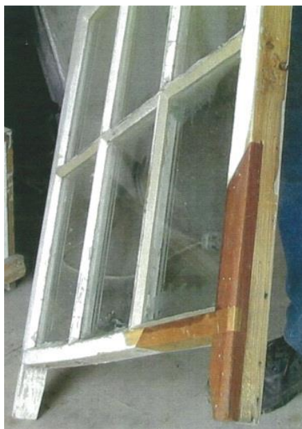
Significant timber framed window repaired with sections of new timber fabric cut into the frame where it had deteriorated. Source: Brian Benson, Ballarat.
