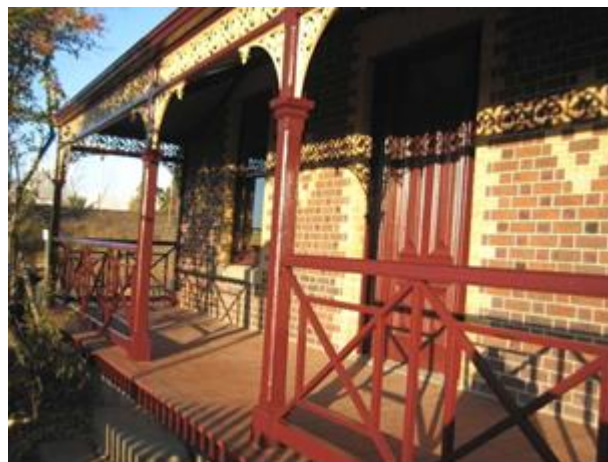
Reconstructed Victorian verandah. The remnant verandah detailing provided clues for the design of the missing cast iron elements, as the surviving detailing was typical of the work of a local 19 th century architect. More intact verandahs known to have been designed by the architect were used to guide the design and detail of missing fabric. Source: Jennifer Bantow.
