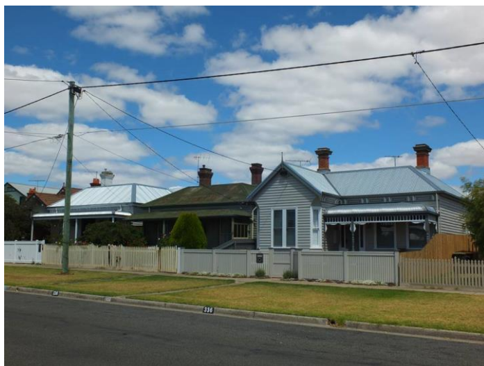
New Zinalume roof cladding (left) and new galvanised steel roof cladding (right). Source: Dr David Rowe.
