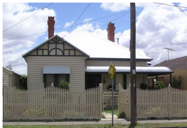
Restored Edwardian dwelling, Geelong West, with reconstructed return verandah and window hood over front window. This represents appropriate replication from a heritage perspective. Source: Dr David Rowe.
