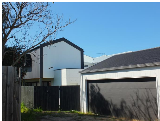
Rear view of two storey additions to the Bungalow, as seen from the lane but not from the principal street. Source: Dr David Rowe.
