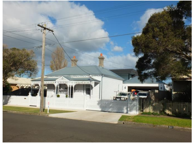
The visibility of the independent two storey additions is incidental (given that it is a separate entity and that does not project directly above or beyond the Late Victorian dwelling). Dr David Rowe.
