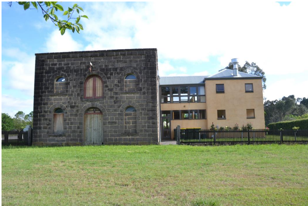
Buangor Stables, Bungaor, Victoria, showing side additions that are recessive and have a lightweight appearance to the strength of the bluestone stables building. Source: Wendy Jacobs, 2018.
