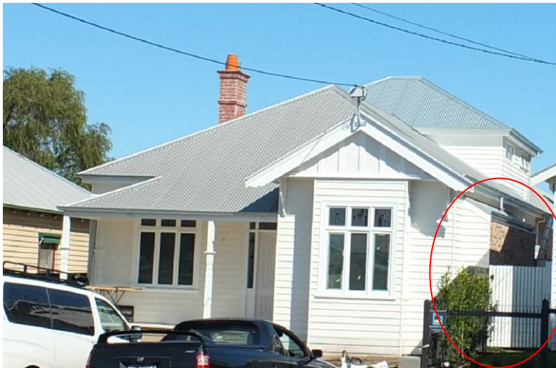
Side ensuite addition located under the eave and set back from the front (circled). Source: Dr David Rowe.
