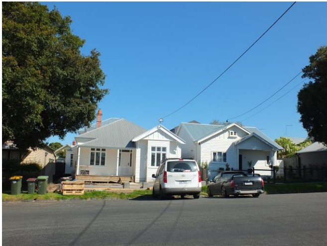
Two storey additions of varying design and construction to the Bungalow (right). The additions are hardly visible from the front. Source: Dr David Rowe.
