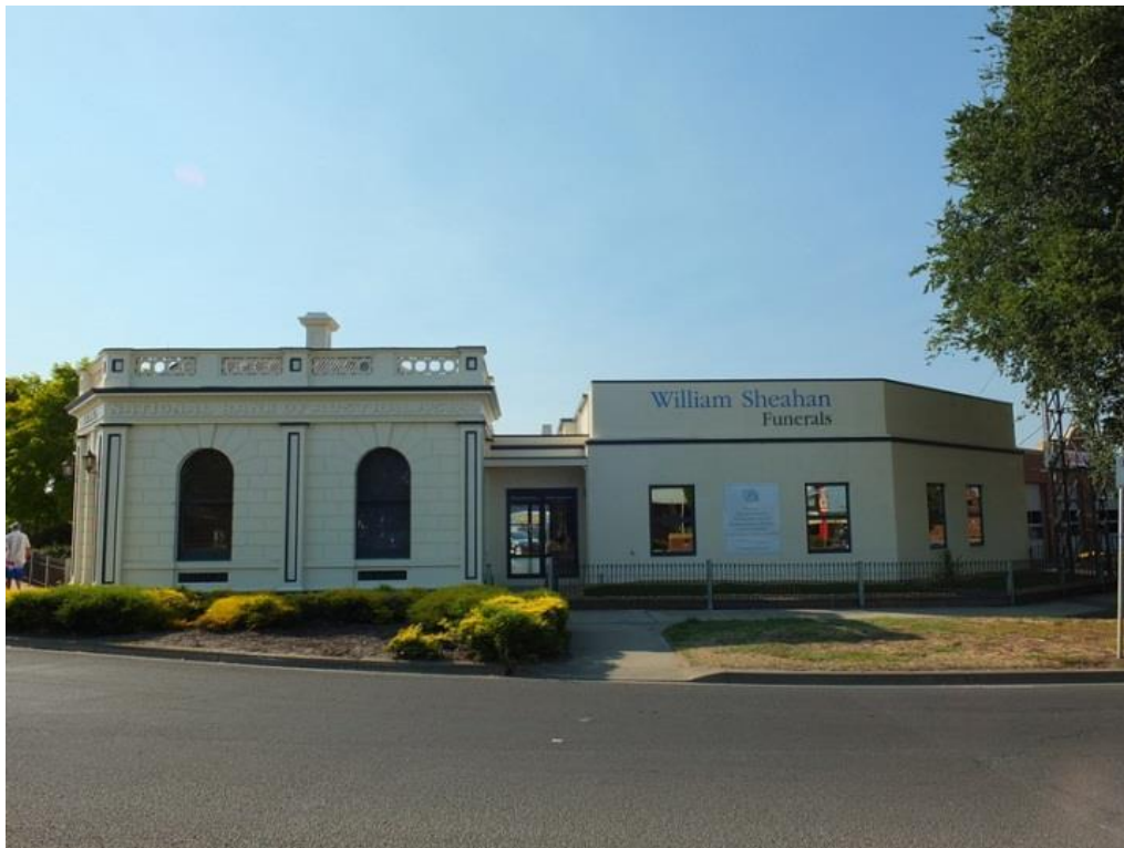
Rear additions connected by a narrow link. The additions are a contemporary interpretation of the heritage asset without being a slavish replica.
