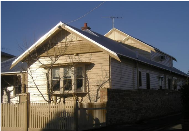
Gabled additions to a hipped and gabled interwar Bungalow. Source: Dr David Rowe.
