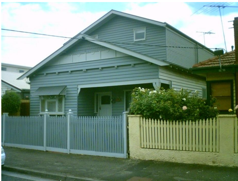
Dominant two storey additions. Source: Dr David Rowe.
