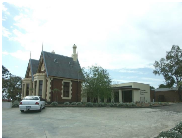
Geelong Eastern Cemetery Gate Lodge with contemporary single storey cuboid additions visible at the rear. Given the subservient proportions 2 and some affinity in the materials between the old and the new, no adverse affect on the significance of the heritage asset has resulted. Source: Dr David Rowe.
