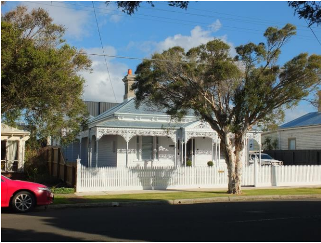
Late Victorian dwelling with rear two storey additions of independent character and yet minimal views from the front. The vertical grey tone has minimise the visual focus of the addition. Source: Dr David Rowe.
