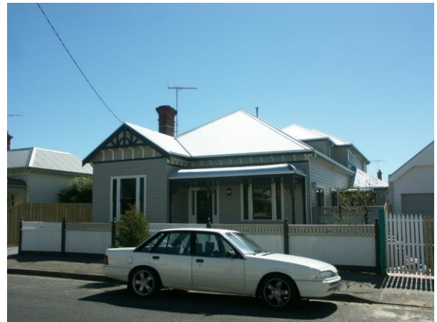
Hipped additions to an Edwardian dwelling where the principal roof form is a hip. Source: Dr David Rowe.
