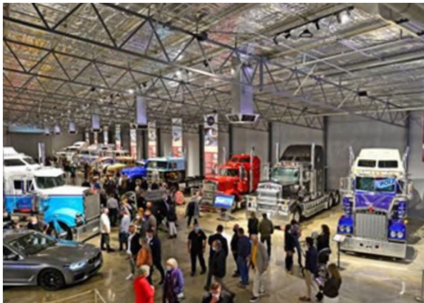
Exposed services with feature lighting to exhibits
