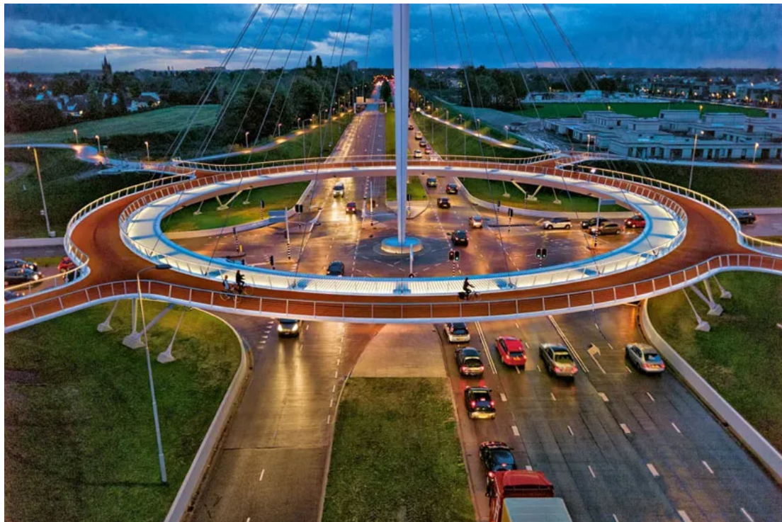
Figure 10 Hovenring: Image source IPV Delft http://www.ipvdelft.nl/
